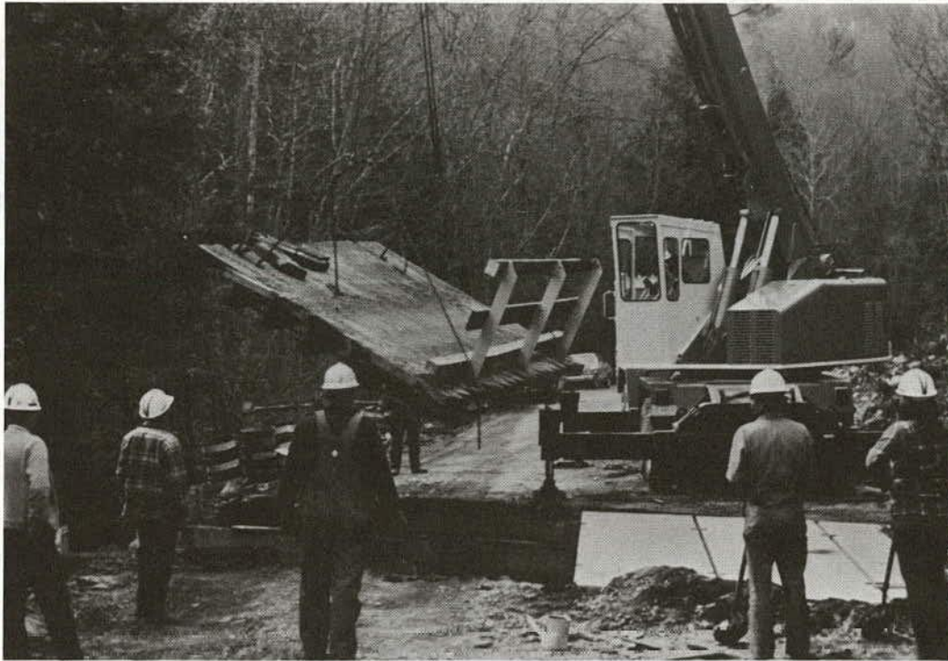
Figure 2 Precast slab spans replace substandard steel stringer-timber deck superstructure (6).
