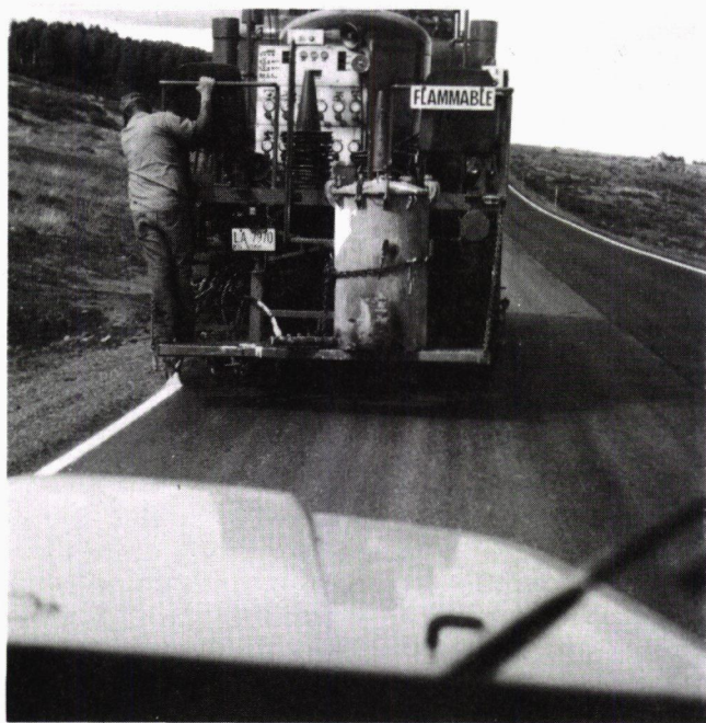
FIGURE 10 Solvent-borne paint-stripping truck.
