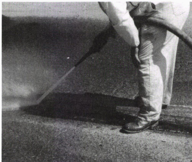
FIGURE 4 Removing chemically reacted markings with a water jet.
