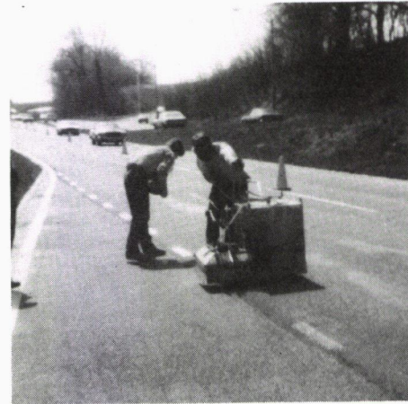
FIGURE 15 Extrusion application of thermoplastic.
