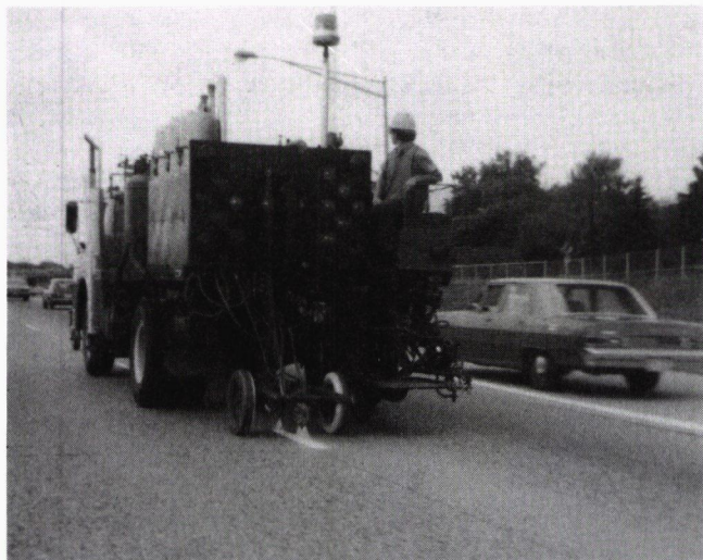
FIGURE 16 Truck-mounted application of polyester pavement-marking material.
