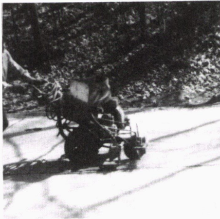
FIGURE 14 Primer being applied prior to application of thermoplastic.
