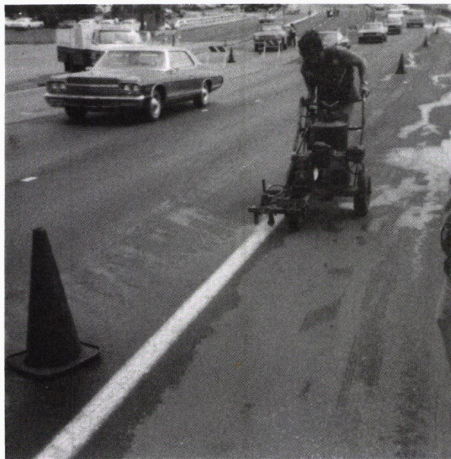
FIGURE 3 Applying chemical removal agent.
