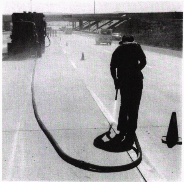
FIGURE 7 Stripe removal with hydroblasting.
