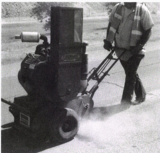
FIGURE 5 Removal of markings by grinding.
