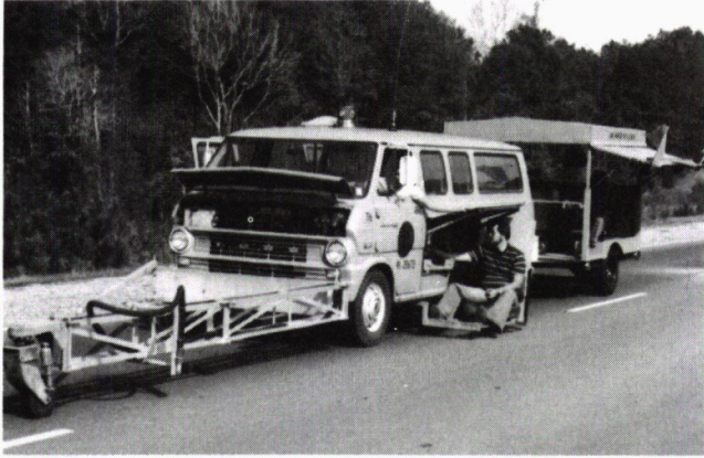
FIGURE 6 Cleaning pavement surface by sandblasting.
