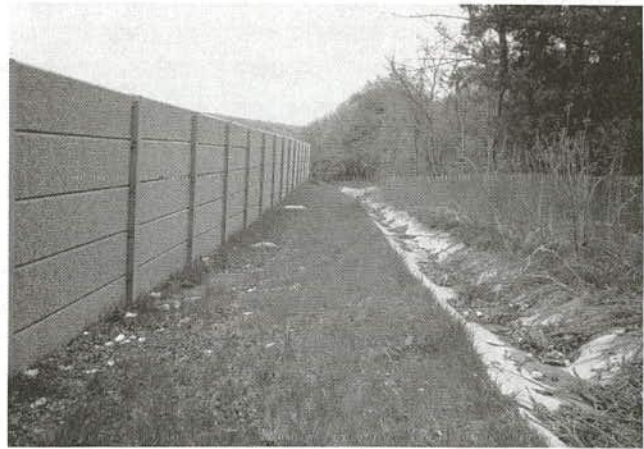
FIGURE D-8 Drainage ditch paved behind sound barrier to facilitate the movement of equipment and reduce drainage problems.
