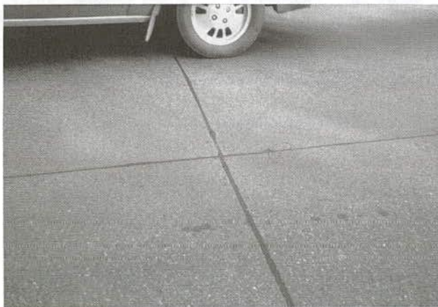
FIGURE D-2 Transverse and longitudinal joints sawed and sealed in overlay on major urban Interstate expressway.
