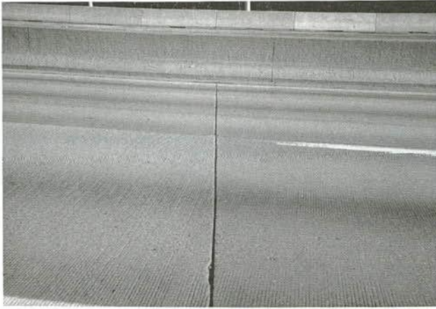
FIGURES D-9 AND D-10 Concrete barrier and shoulders complement a thick unbonded concrete pavement overlay of existing old Interstate in Pittsburgh, Pa. Preformed joint seals were also used to reduce the need for future maintenance.
