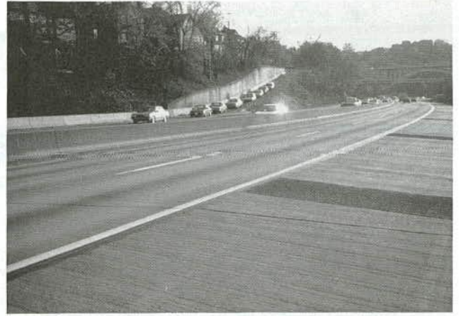
FIGURES D-9 AND D-10 Concrete barrier and shoulders complement a thick unbonded concrete pavement overlay of existing old Interstate in Pittsburgh, Pa. Preformed joint seals were also used to reduce the need for future maintenance.
