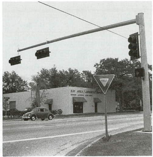
FIGURE 32 Monotube mast arm assembly.
