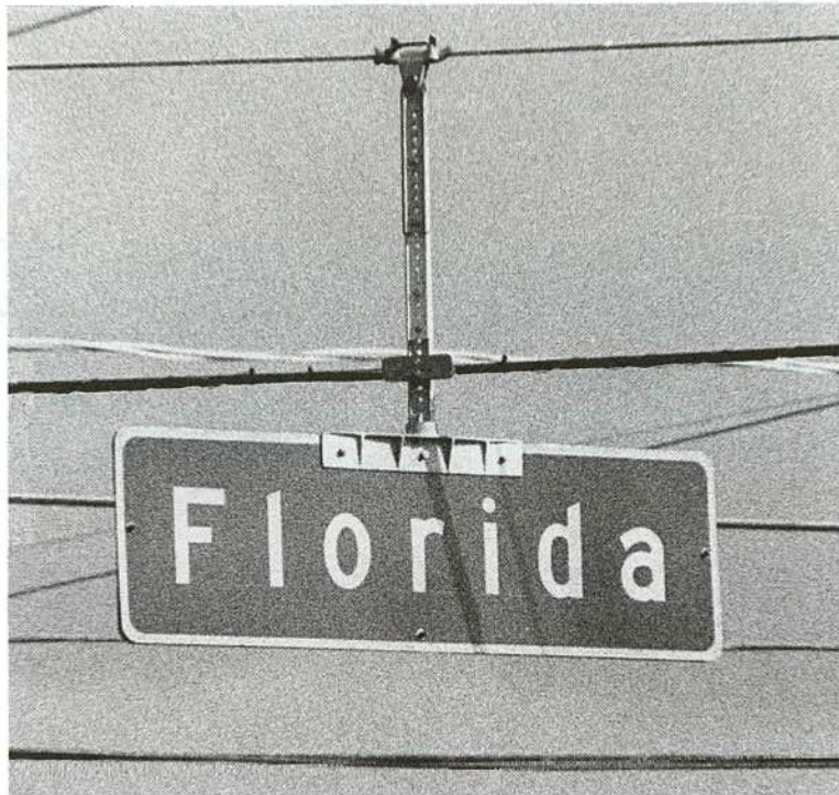
FIGURE 36 Overhead street name sign.
