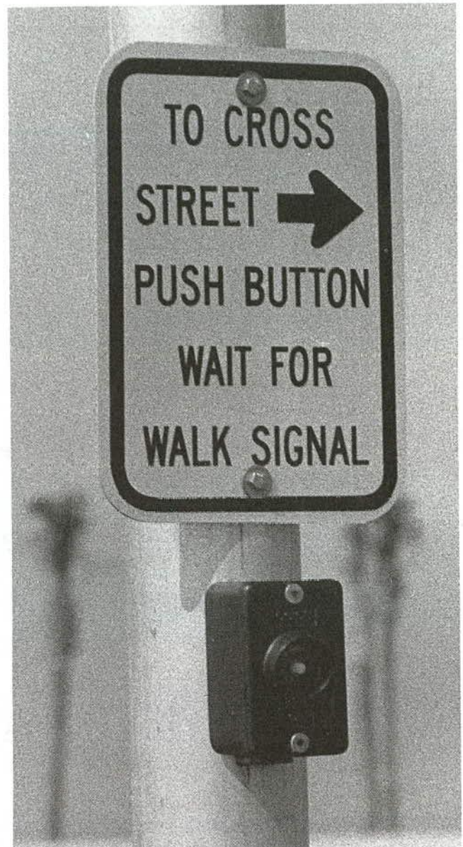
FIGURE 18 Pedestrian push button.
