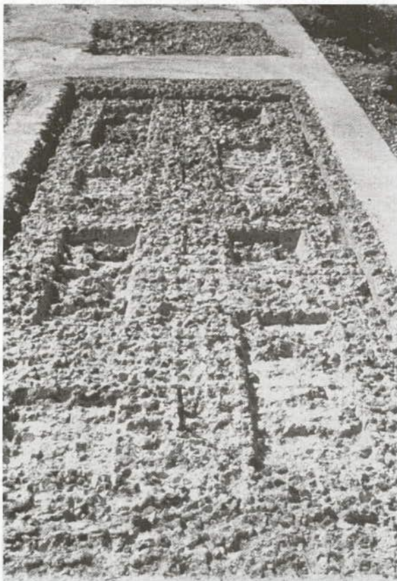
FIGURE 13 Use of hydrodemolition to remove weak concrete.
