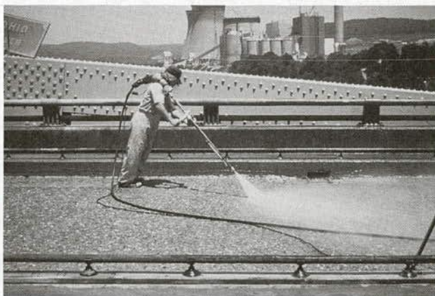
FIGURE 22 A waterblasting operation.
