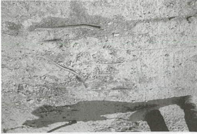
FIGURE 19 Effect of using a scarifier in an area of low cover.
