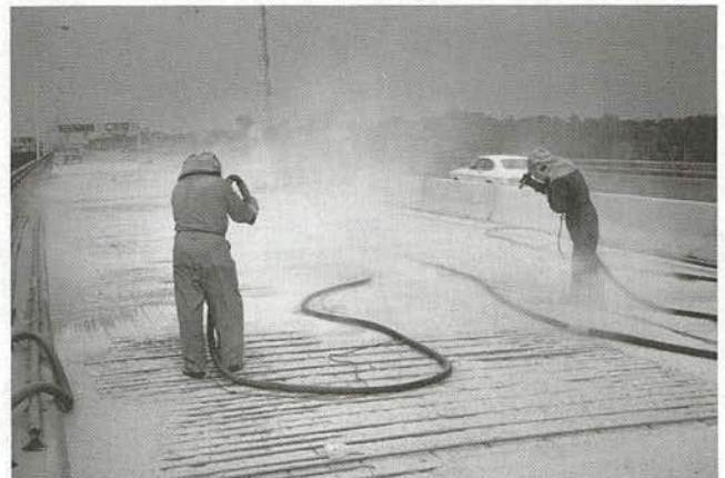
FIGURE 20 A typical sandblasting operation.
