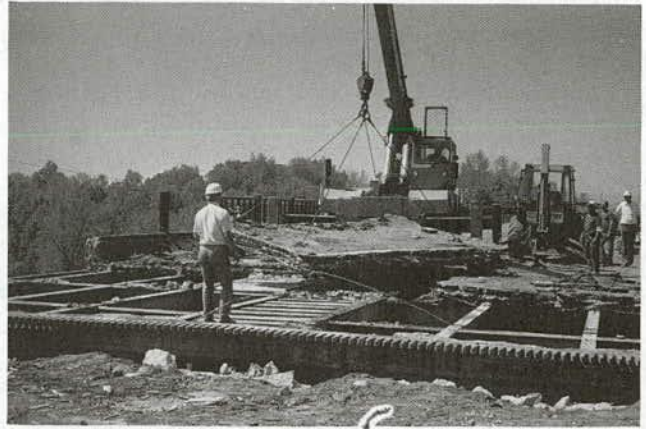
FIGURE 4 Use of a crane to remove a section of deck slab.
