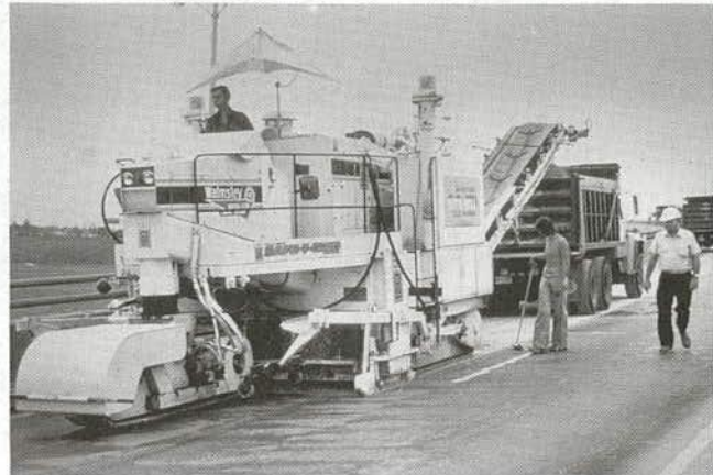
FIGURE 17 A large scarifier with a conveyor to remove scarified concrete.
