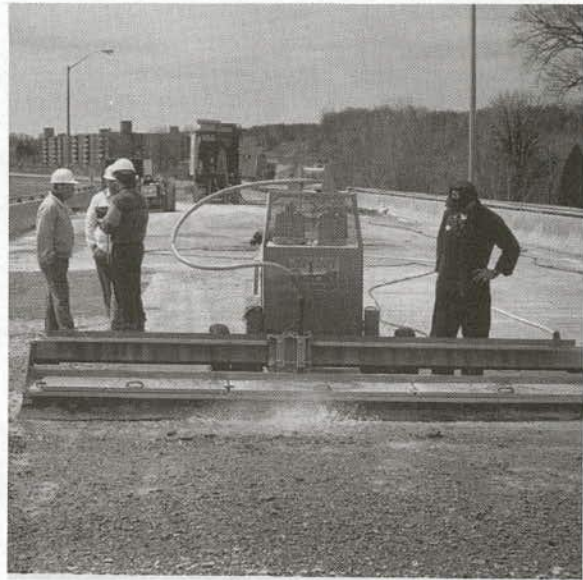
FIGURE 14 A commercial hydrodemolisher.
