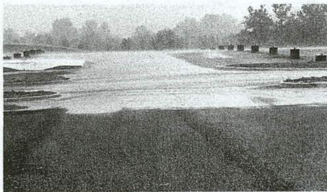
FIGURE 31 Porous pavement (foreground) compared with conventional pavement (background) during a storm.
