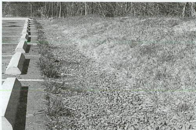
FIGURE 28 An infiltration trench at a parking lot.
