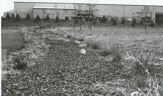
FIGURE 50 Infiltration trench with long vegetative buffer strip.
