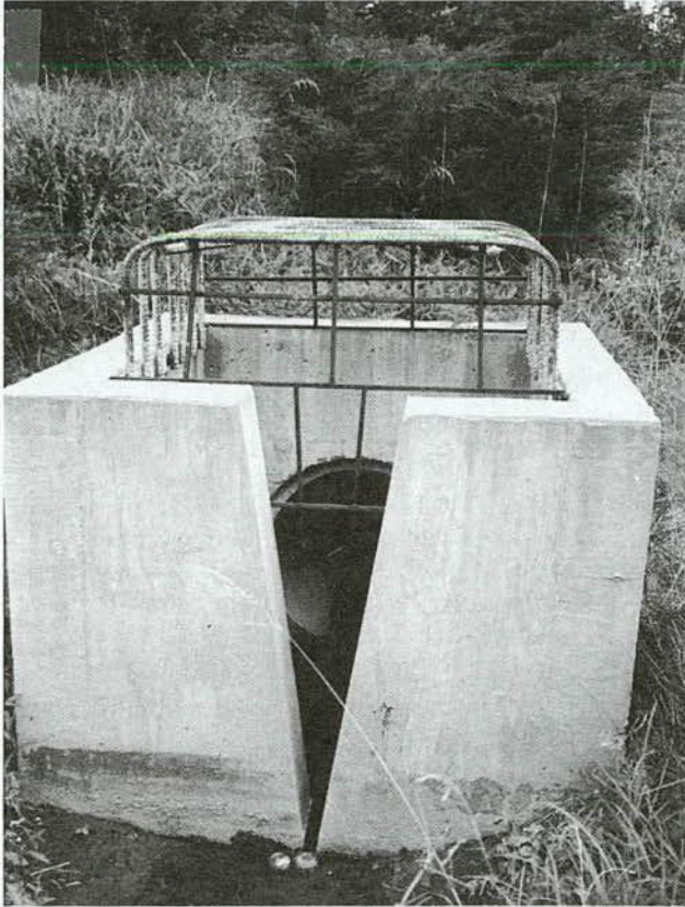
FIGURE 42 Extended dry pond outlet design (photo by R. Kaign).
