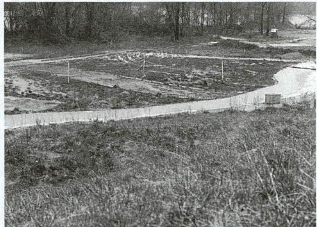
FIGURE 32 Level spreader/vegetative filter strip system (86).
