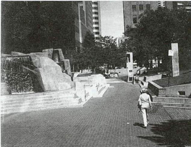
FIGURE 19 Depressed parkway in downtown Denver, CO; multiple-purpose use, passive recreation and stormwater storage. (Photo courtesy of Urban Drainage and Flood Control District, Denver, Colorado.)
