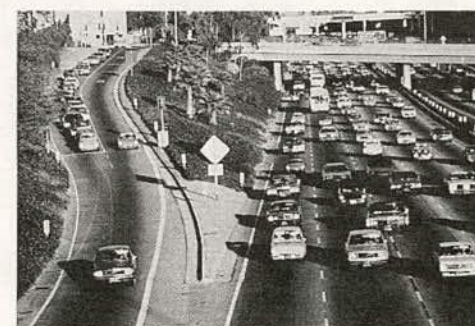
Ramp meter bypass, I-10, Los Angeles (photo: California DOT)
