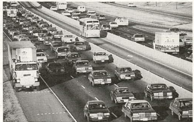
Katy transitway was constructed in the freeway median in 18 months
