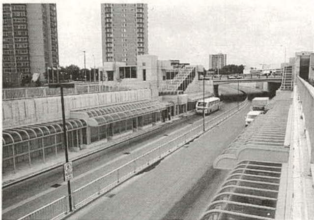
On-line transit station, Ottawa, Canada
