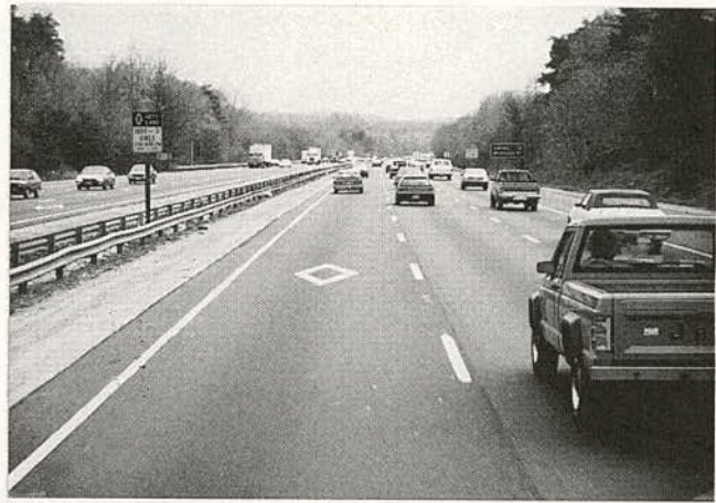
I-95 interim HOV lane, northern Virginia
