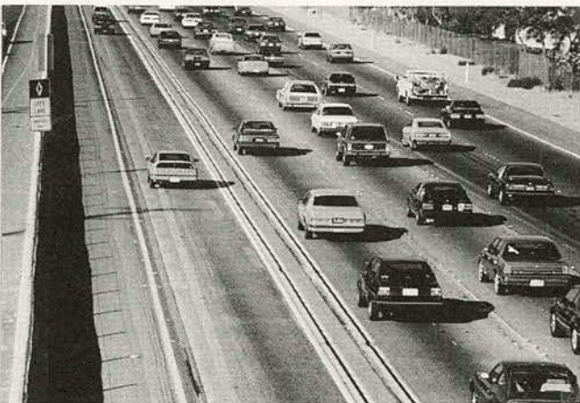
FIGURE 9 Typical concurrent-flow, buffer-separated facility (SR 55, Orange County, California).
