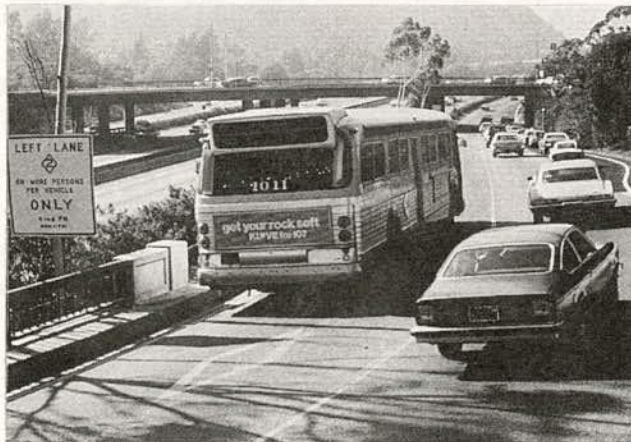
FIGURE 12 Typical HOV queue bypass (I-10 metered freeway entrance ramp, Los Angeles).
