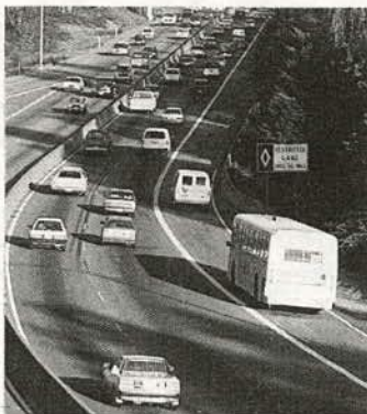
SR 520 bus bypass
