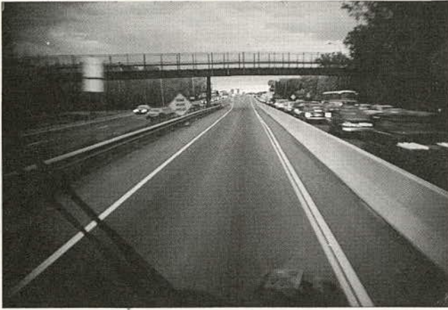
Reversible-flow lane during construction of two-lane reversible-flow
