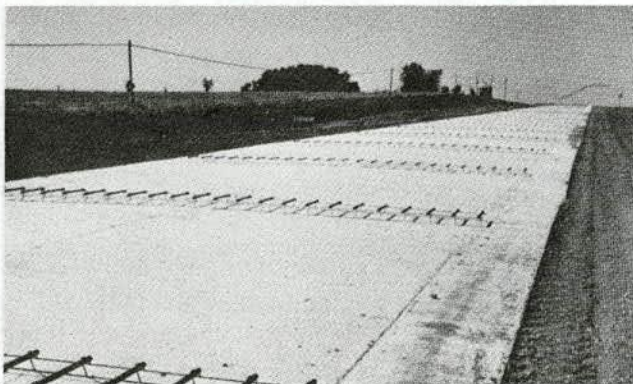
FIGURE 17 Dowel assemblies in place prior to paving (9).
