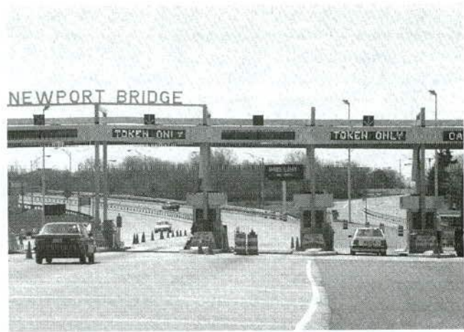
FIGURE 28b Canopy-mounted VMSs used to designate lane status and method of toll collection, Newport Bridge toll plaza, Rhode Island (Fiberoptic Display Systems, Smithfield, Rhode Island).
