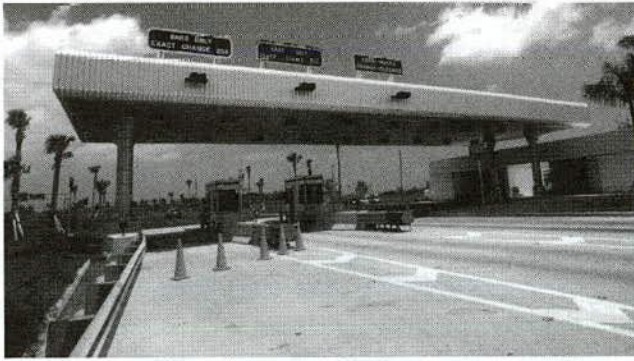
FIGURE 21a Metal-clad canopy, Florida Turnpike ramp toll plaza (Parsons Brinckerhoff, New York).
