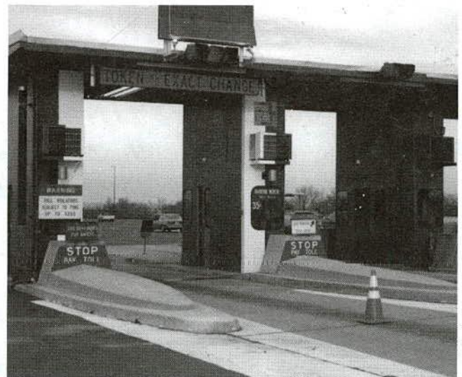
FIGURE 27c Flip signs above and below canopy, Garden State Parkway (New Jersey Highway Authority).
