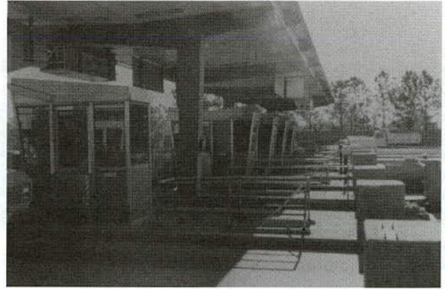
FIGURE 10 Typical toll island tunnel stairwells, former Norfolk-Virginia Beach Expressway. Stairwells are located on every other island.
