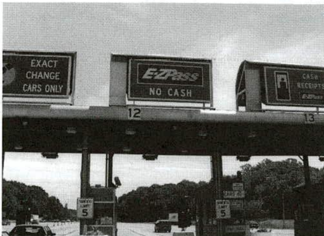
FIGURE 27a Canopy-mounted changeable message signs designate collection methods available in lanes, New York State Thruway Spring Valley toll plaza (New York State Thruway Authority).
