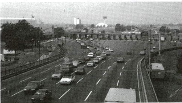
FIGURE 6 Example of a one-way toll conversion, Walt Whitman Bridge toll plaza, Philadelphia, Pennsylvania. Tolls are collected in the direction of oncoming traffic in the photo; traffic going in the other direction pays no toll (congestion due to bridge construction).
