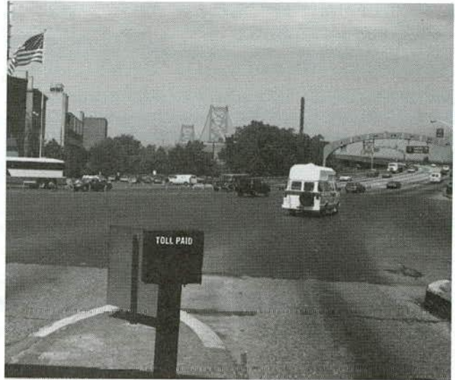
FIGURE 22 Patron fare indicator (PFI), Benjamin Franklin Bridge toll plaza, Camden, New Jersey (Delaware River Port Authority).
