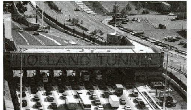
FIGURE 21d Overhead utility rooms and toll lane access, Holland Tunnel toll plaza (Port Authority of New York and New Jersey).
