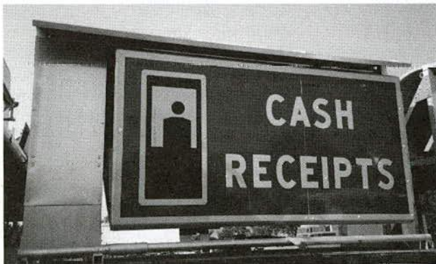
FIGURE 9a Canopy-mounted changeable message sign, Tappan Zee Bridge toll plaza. Symbols, colors, and legends are used to inform motorists of lane payment methods (New York State Thruway).
