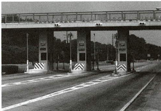
FIGURE 21c Pedestrian walkway over canopy, Chesapeake Bay Bridge-Tunnel toll plaza, Virginia.
