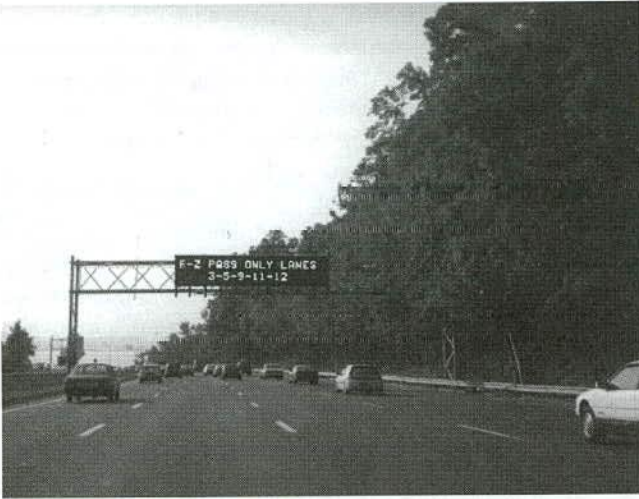
FIGURE 28a Advance variable message sign (VMS) designating available ETC lanes (E-ZPass), Tappan Zee Bridge, Nyack, New York (New York State Thruway Authority).
