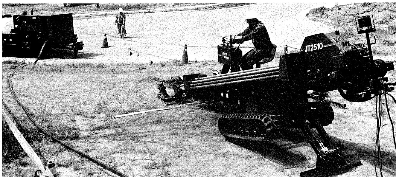
FIGURE 1 Conduit being installed under a roadway with a trenchless installation method.
