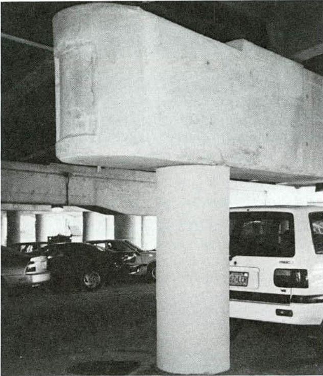
FIGURE 37 FRP wrapped column.
