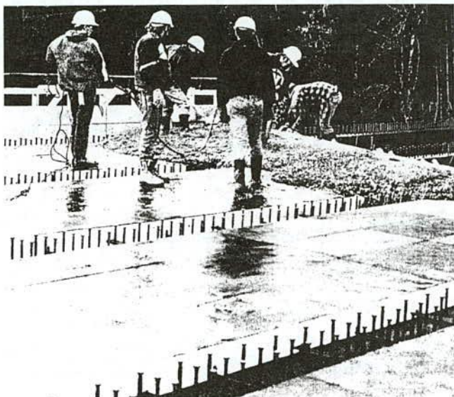
FIGURE 40 Placing FRC deck, Salmon River Bridge (157).
