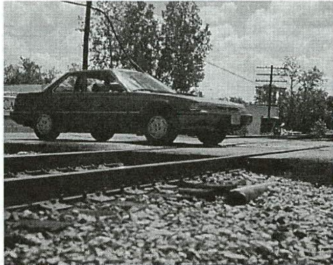
FIGURE 14a A properly drained crossing surface.
