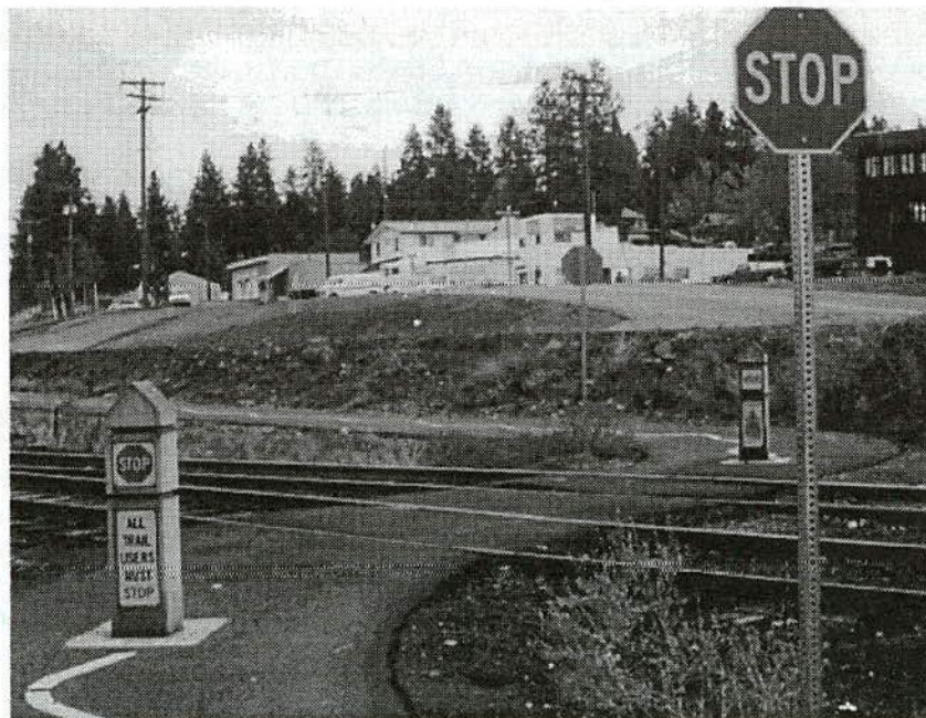
FIGURE 16 Relocated bike path to elevate bad-angle crossing.
