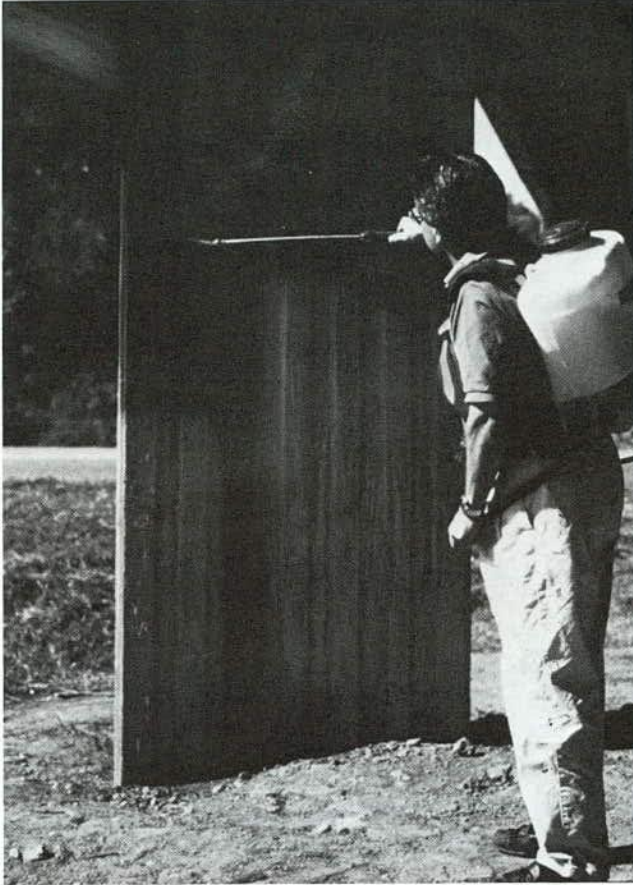
FIGURE 13 Cleaning rust stains.
