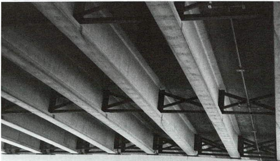
FIGURE 14 Weathering steel diaphragms with prestressed beams.
