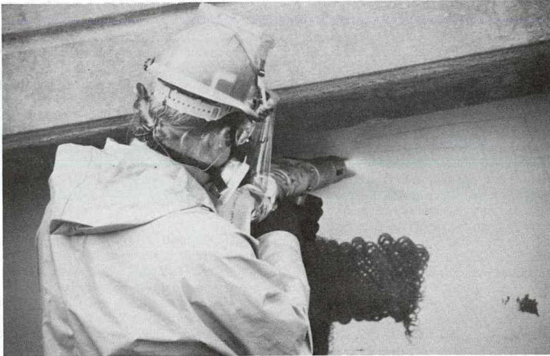
FIGURE 19 Ultrahigh pressure water jetting.
