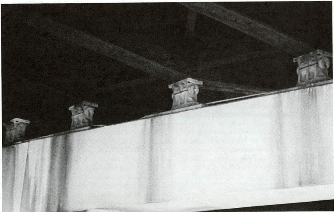
FIGURE 11 Installed galvanized bearing.
