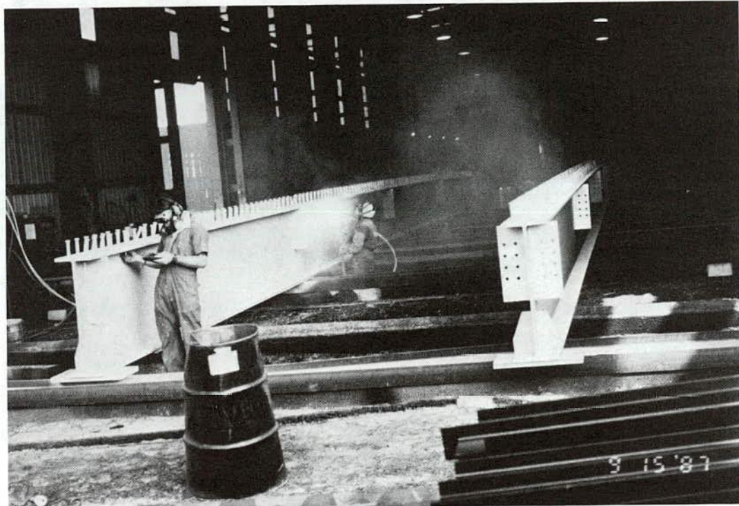
FIGURE 8 Electric arc metallizing in shop.
