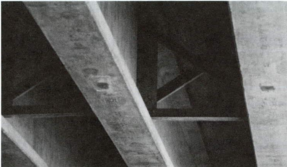
FIGURE 24 Cross-bracing diaphragms.
