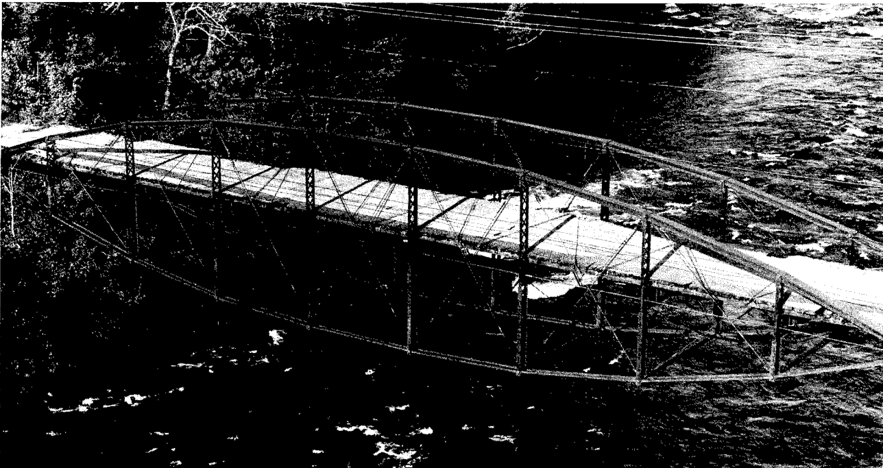
FIGURE 3 Old Corinth Road Bridge over the East Branch of the Sacandaga River, Hadley, New York (photo credit: Jet Lowe).
