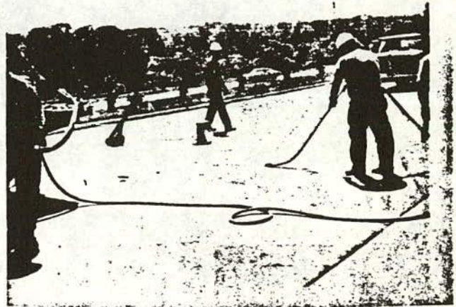
Fig 5 5-791.074 - Blow joint with air after sandblasting. Note hook on end of air hose pipe; this is used to aid in removal of rocks stuck in joint. If sliver of concrete is present, remove at this time.
