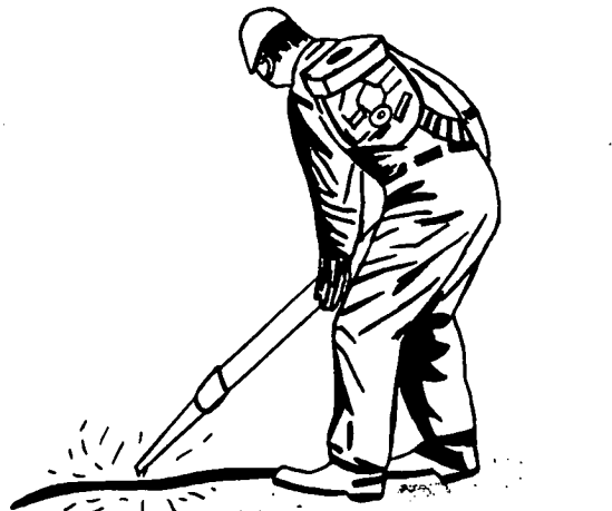
FIGURE 7 Cleaning joint with air.
