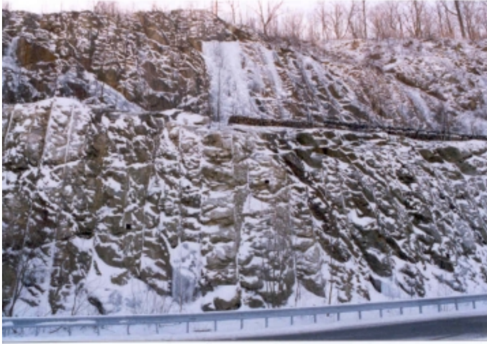
Figure 6-3: Rock Bolts Observed Along NYS Route 9W, Hudson Highlands.
