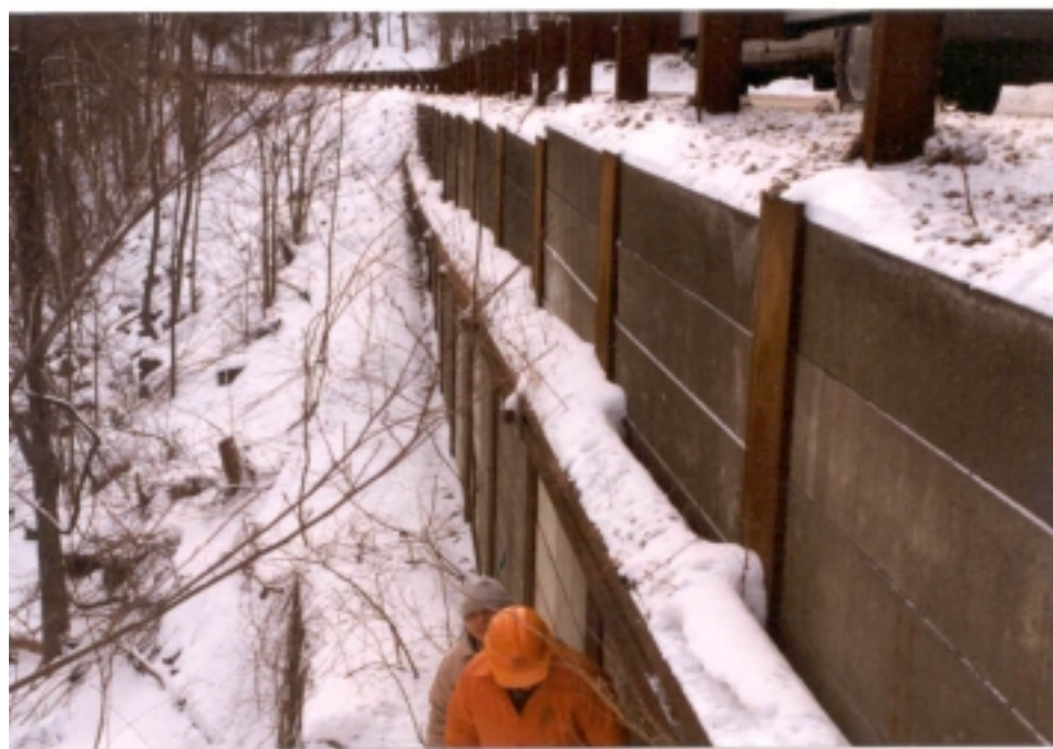
Figure 6-8: Soldier Pile and Lagging Wall, Palenville, NY.
