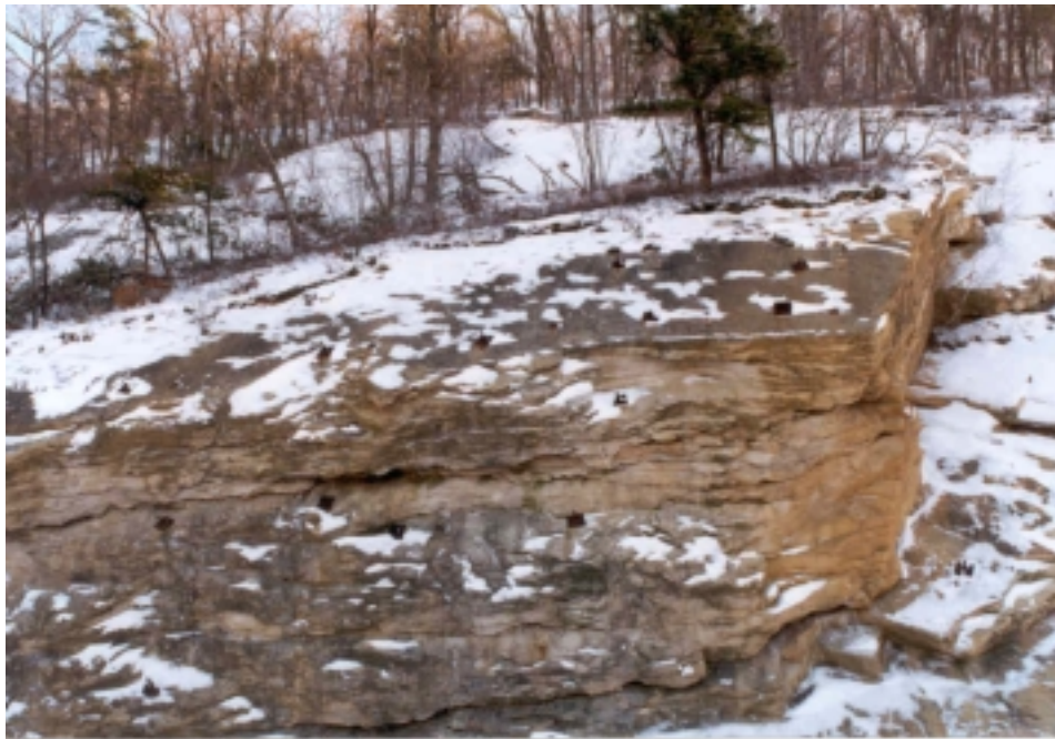
Figure 6-2: Rock Bolts Observed Along NYS Route 52 in Ellenville, NY.
