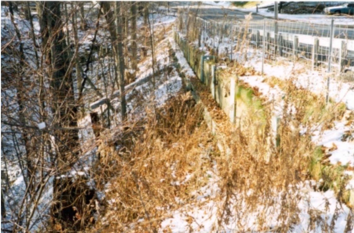
Figure 6-9: Soldier Pile and Lagging Wall, Gawanda, NY.
