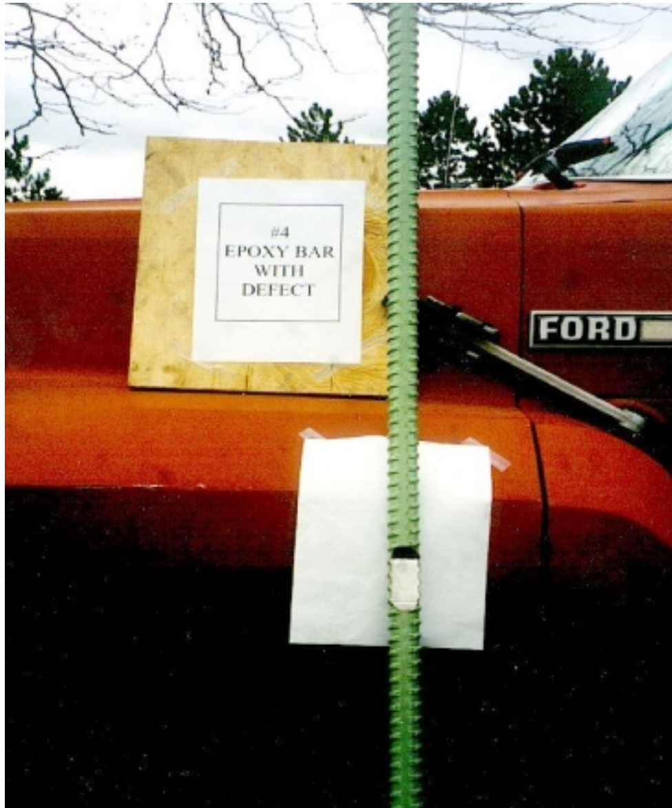
Figure 3-6(c): In-Situ Specimen #4: Epoxy Bar With Defect.
