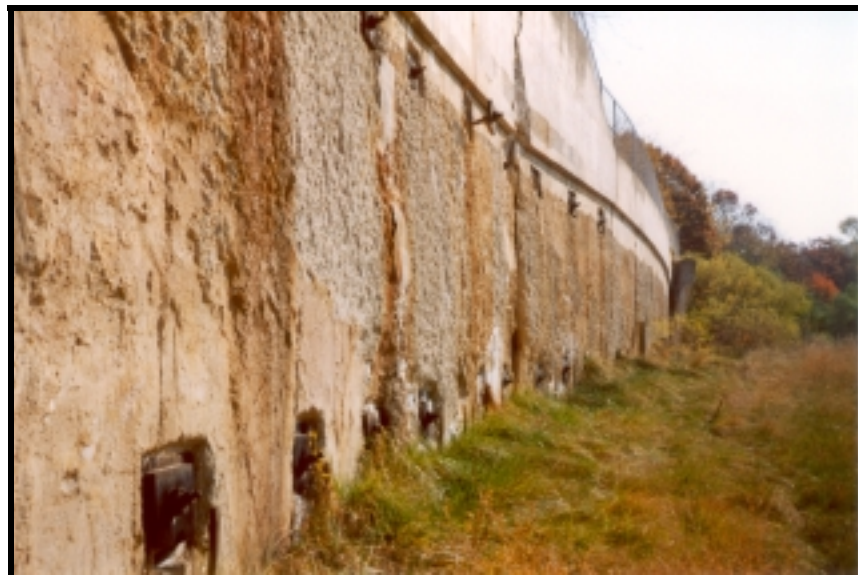
Figure 6-7: Anchored Concrete Diaphragm Wall, Washington, DC.
