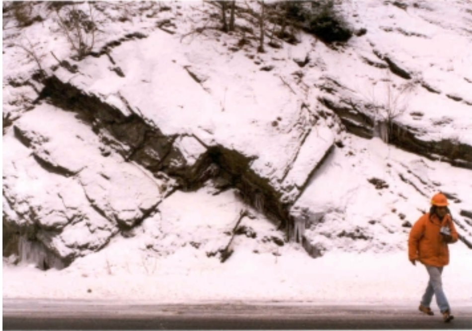
Figure 6-1: Rock Bolts Observed Along NYS Route 22.
