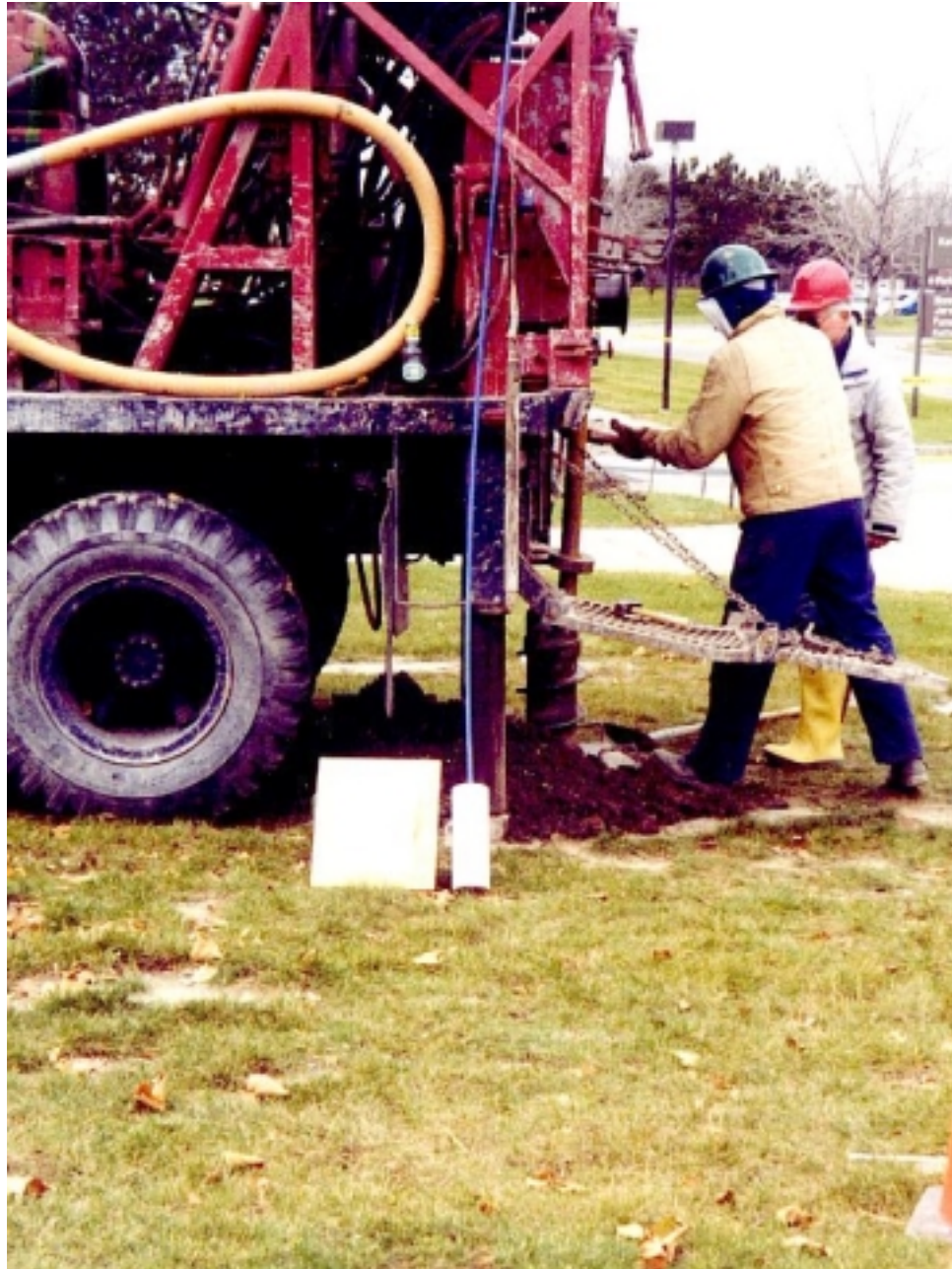
Figure 3-3: Installation of In-Situ Specimens.
