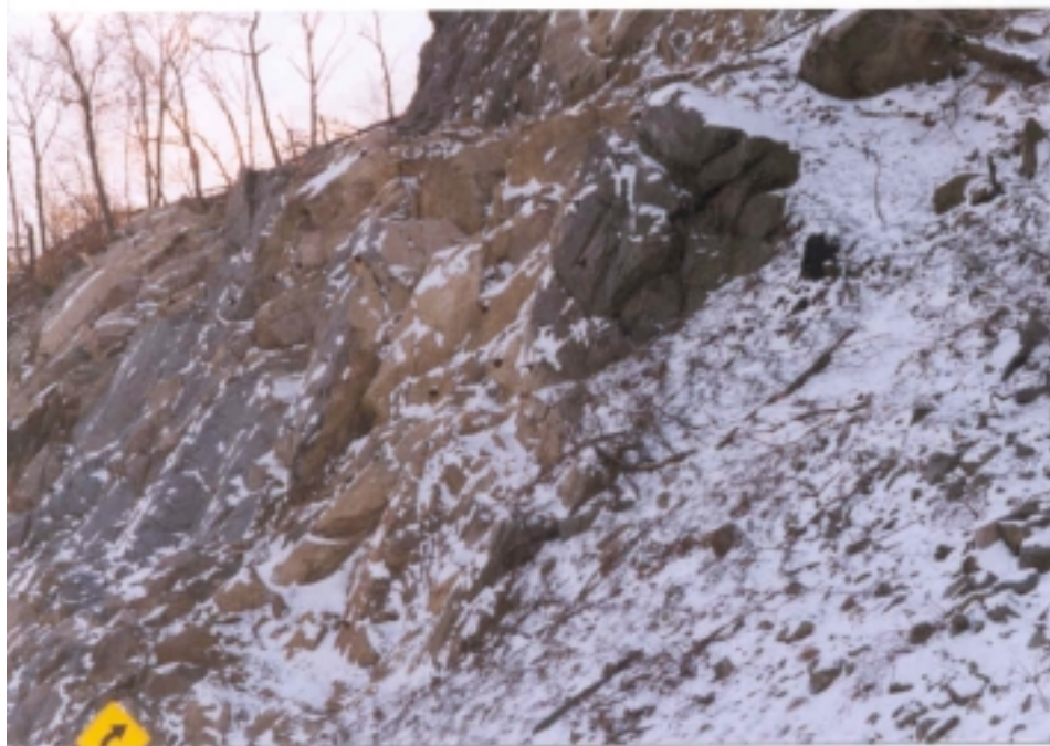
Figure 6-4: Rock Bolts Observed in Bear Mountain State Park, NY.
