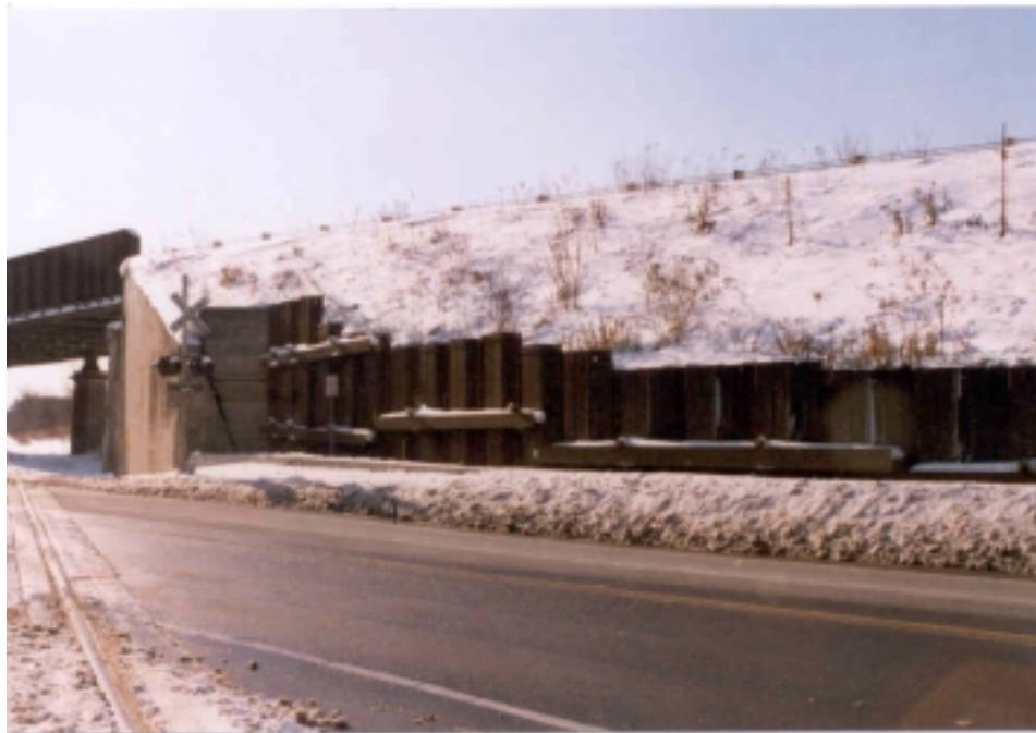
Figure 6-10: Tied-Back Wall for Embankment, Conrail Over NYS Route 5.
