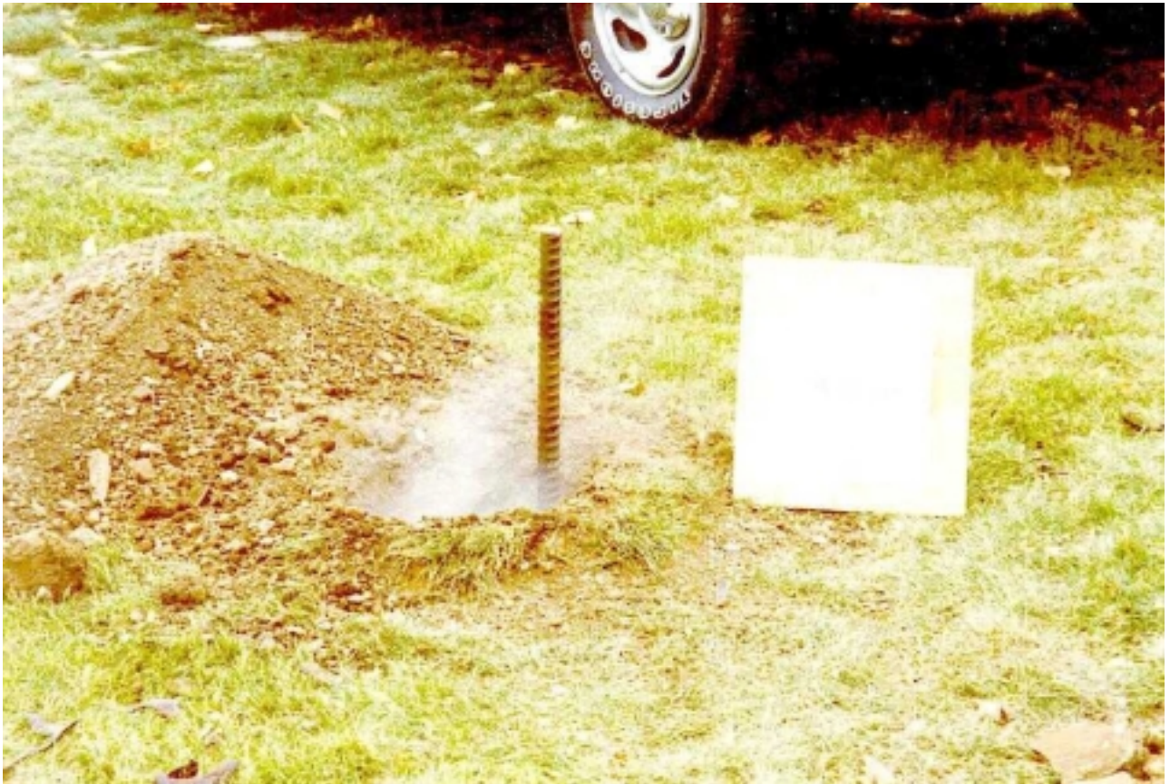
Figure 3-6(a): Installed In-Situ Specimen #1: Plain Bar.
