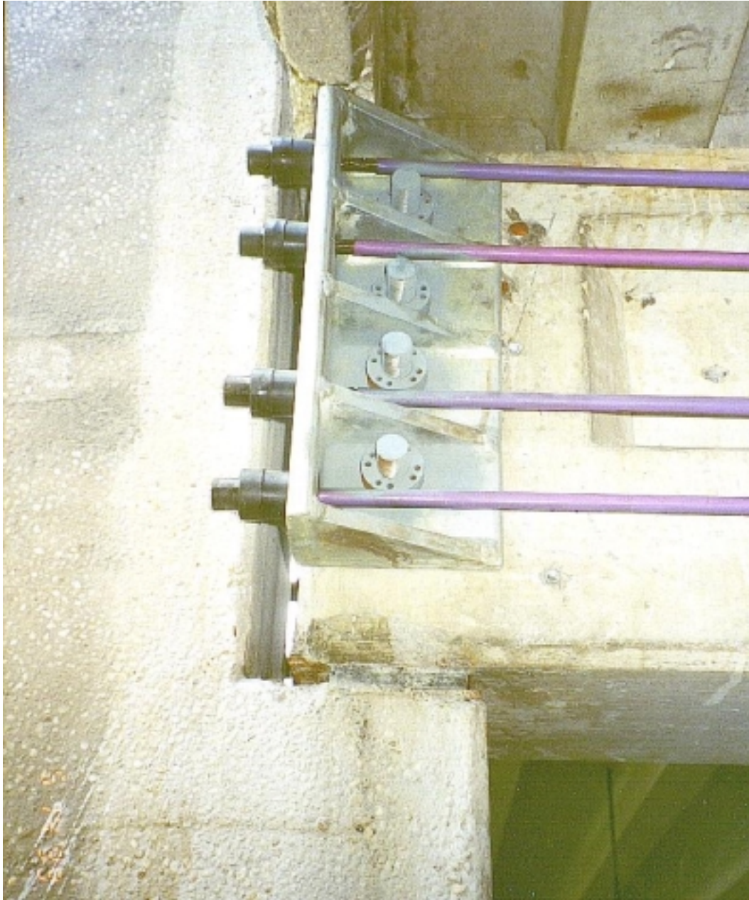
Figure 3-12(b): Tendon Anchorage at Niagara Falls Parking Garage.
