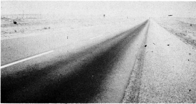
Figure 14. An asphaltic-concrete surface with flushing in the outside lane, outside lane coefficient = 0.39 and inside lane coefficient = 0.55, age = 3 yr, ADT = 6210, basalt, 60 percent fractured faces, 5.75 percent asphalt content.
