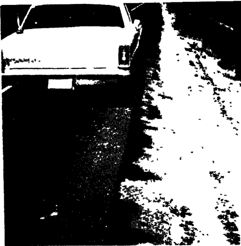
Figure 12. Good surface drainage from a plant-mix seal.
