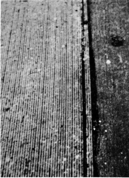
Figure 20. A concrete surface with longitudinal grooving on the left and the original surface on the right; coefficient on grooved section (left) = 0.40 and coefficient on ungrooved section (right) = 0.35, age = 15 yr, ADT = 2850 (other information not available).
