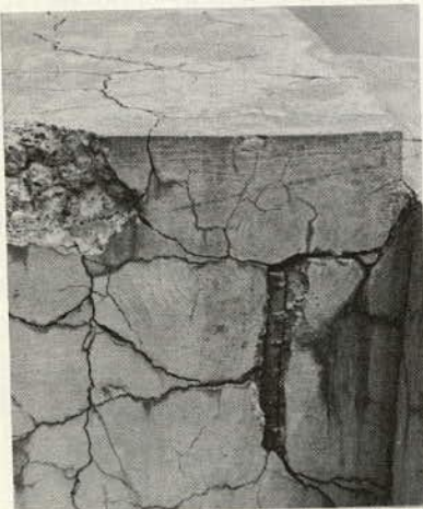
Figure 6. Hand rail post in 1956 (left) and 1964 (right) vertical expansion is 1 \frac{3}{16} in. in spite of reinforcing.
