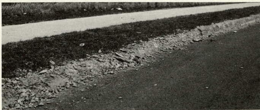
Figure 1. Close-up of section of a deteriorated concrete curb, affected area.
