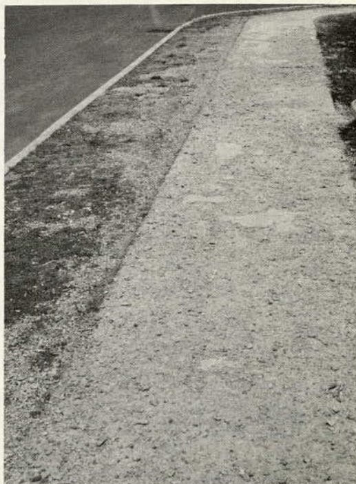
Figure 2. Deteriorated concrete sidewalk, affected area.
