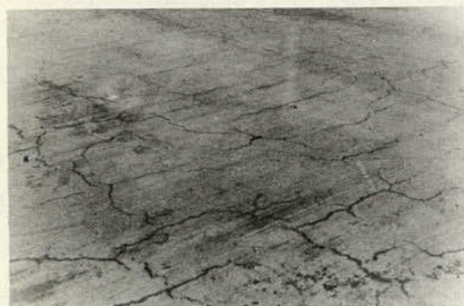
Figure 1. Random cracking in span 4 (surface damp).
