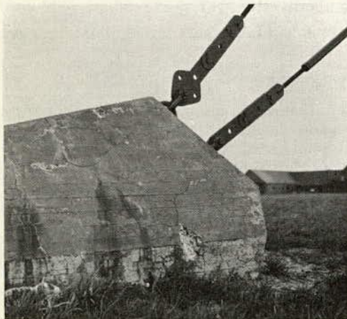
Figure 1. Anchorage block 8 (Fig. 2) with coarse cracks and map-cracking.
