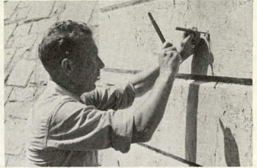
Figure 4. Setting brass insert with lead wool. This concrete is expanding at 0.03 percent per year.
