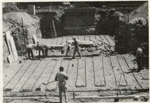
Figure 7. Wrought iron coils on sand backfill in heat exchanger 2.
