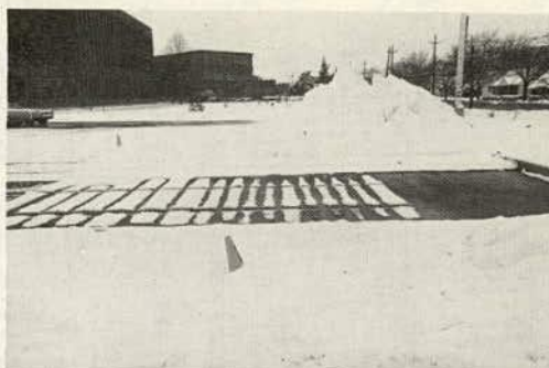
Figure 12. Panel 1 at 1:15 p.m. on January 7, 1970—pipes on 6-, 12-, and 18-in. centers.
