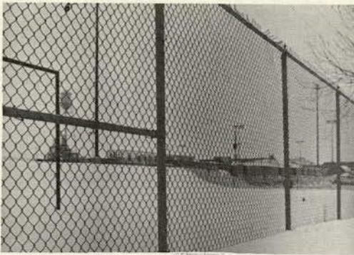
Figure 5. A steel wire fence is not very effective as a windbreak or snow barrier.
