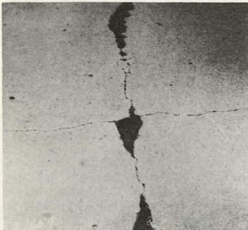
Figure 7. Maintenance on longitudinal crack.
