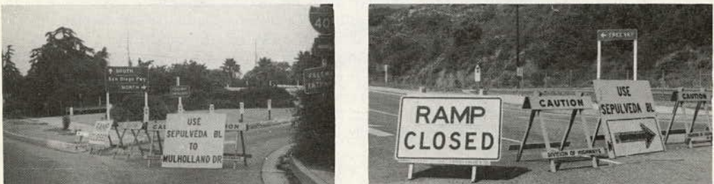
Figure 6. Ramp closures and alternate route signs.
