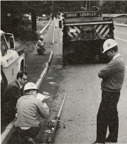
Figure 2. Measurement of pavement deflection and rebound using Benkelman beam.
