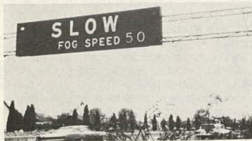
Figure 5. Changeable-message sign on I-5 in Oregon will be controlled by Videograph.
