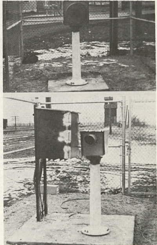
Figure 4. Skopograph projector and receiver monitors visibility at Commonwealth Edison's Dresden Power Station at Morris, Illinois.
