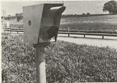
Figure 3. Videograph on Pennsylvania Turnpike, east of Carlisle, controls strobe lights in experimental lighting program.
