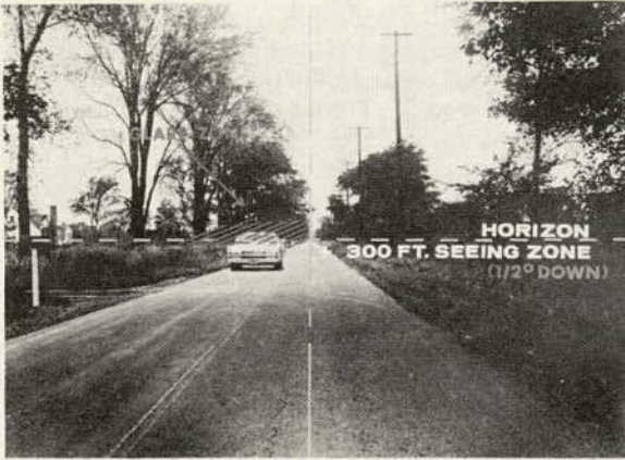
Figure 2. Vehicle encounter lighting problem.
