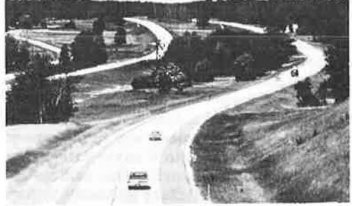
Figure 2. Long reverse curves enhance the driver's view and eliminate the monotony of long tangents.
