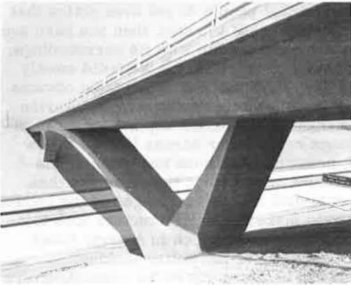
Figure 1. Miramar Road overcrossing near San Diego.
