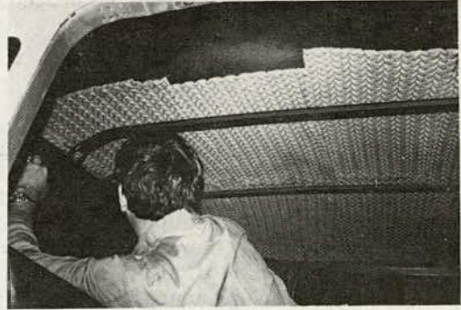
Figure 4. Installation of acoustic headliner.
