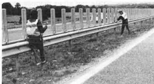
Figure 8. Close-up of attachment of vanes to tensioned safety fence.
