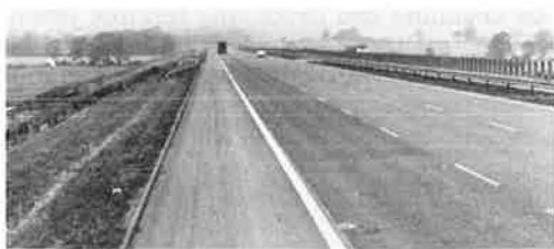
Figure 7. Experimental antiglare fence.
