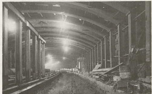
Steel supports in tunnel (photo courtesy of Commercial Shearing, Inc.).
