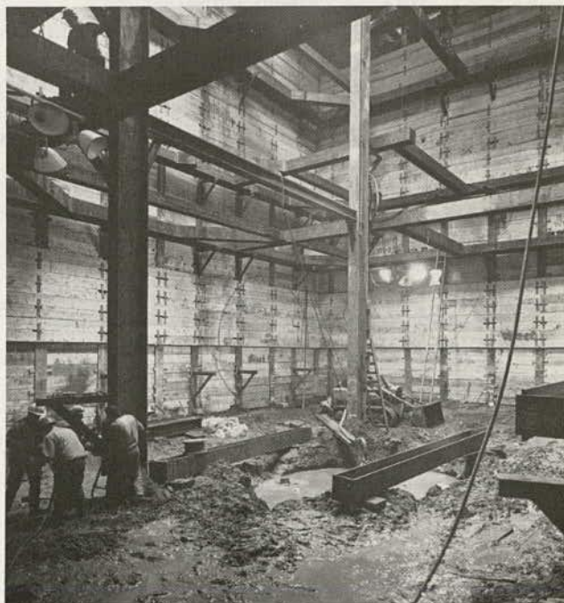
Excavation bracing for subway station.
