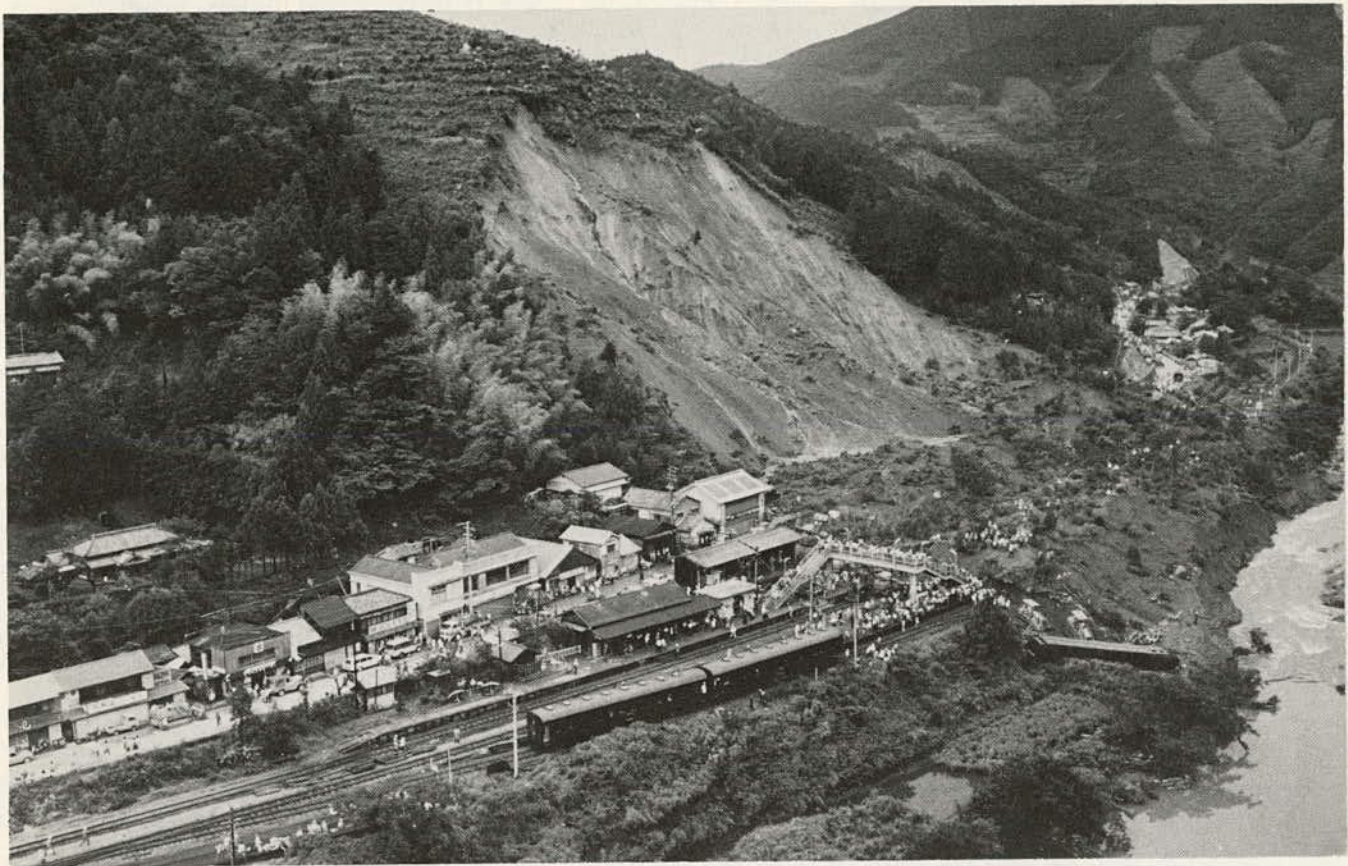
Figure 1.3. Damage to railway facilities from 1972 Segeto landslide in Japan.
