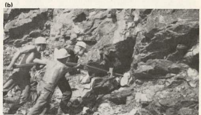
Figure 9.35. Installation of system shown in Figure 9.34: (a) location of two benches where the trial anchor installation is conducted, (b) inserting the cable in the borehole, (c) formwork for horizontal concrete stringer on lower bench and 66-44 welded wire mesh, (d) formwork for anchor pads on top bench and steel bar horizontal stringer, (f) cable anchor tensioned and locked, and (f) completed trial anchor installation on lower bench (9.4).
