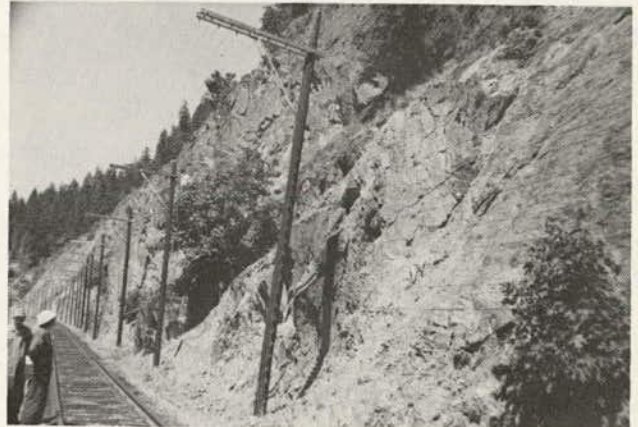
Figure 9.58. Standard type of railway electric warning fence with wires strung between upright poles and horizontal members that are cantilevered out from top of poles along Canadian National Railway line in Fraser Canyon, British Columbia.
