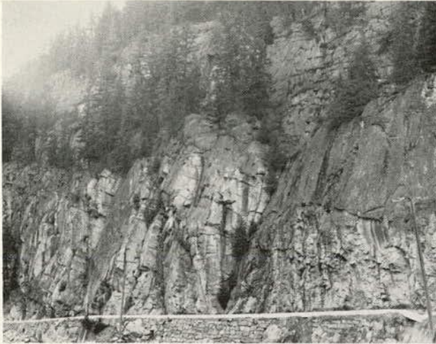
Figure 9.2. Well-developed discontinuities dipping toward highway at Porteau Bluffs, British Columbia. Two significant slides have occurred in this area.
