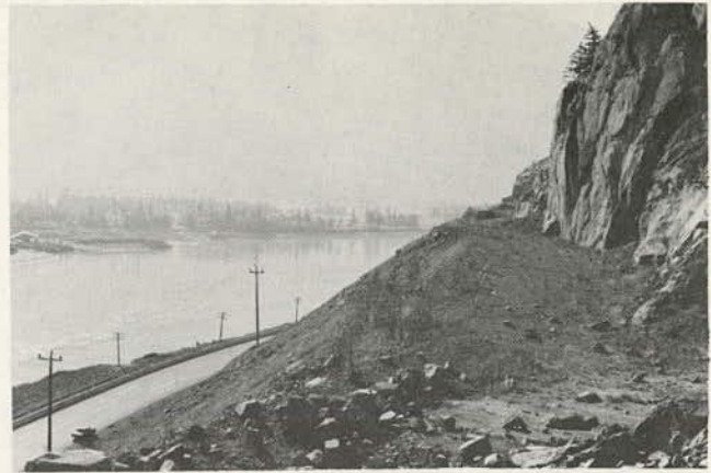
Figure 9.42. Shaped berm that is at toe of high rock face and cut in top of high talus slope above Hope-Agassiz highway in British Columbia.
