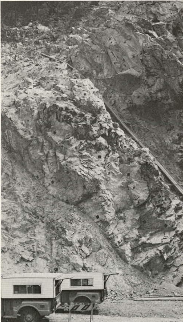
Figure 9.30. Broadly distributed 1.6-cm ( \frac{5}{8} -in) diameter by 1.2 to 3-m (4 to 10-ft) long rock bolts at Hell's Gate Bluffs, British Columbia. These rock bolts were posttensioned to about 53.4 kN (6 tf) to maintain integrity of small individual blocks in slope.
