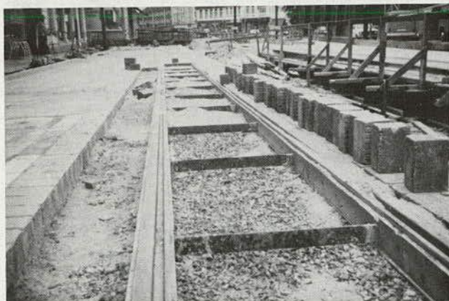
Figure 2. Construction of resilient track in Heissen in 1975 (ballast base, block pavement).
