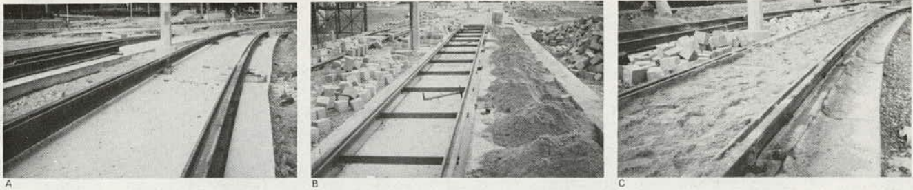
Figure 9. Construction of slab-based-block paved track.
