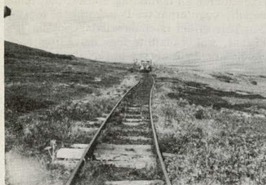
Figure 3. Roadbed of Seward Peninsula Tramway Displaced by Movement of Active Lobate Terrace.
