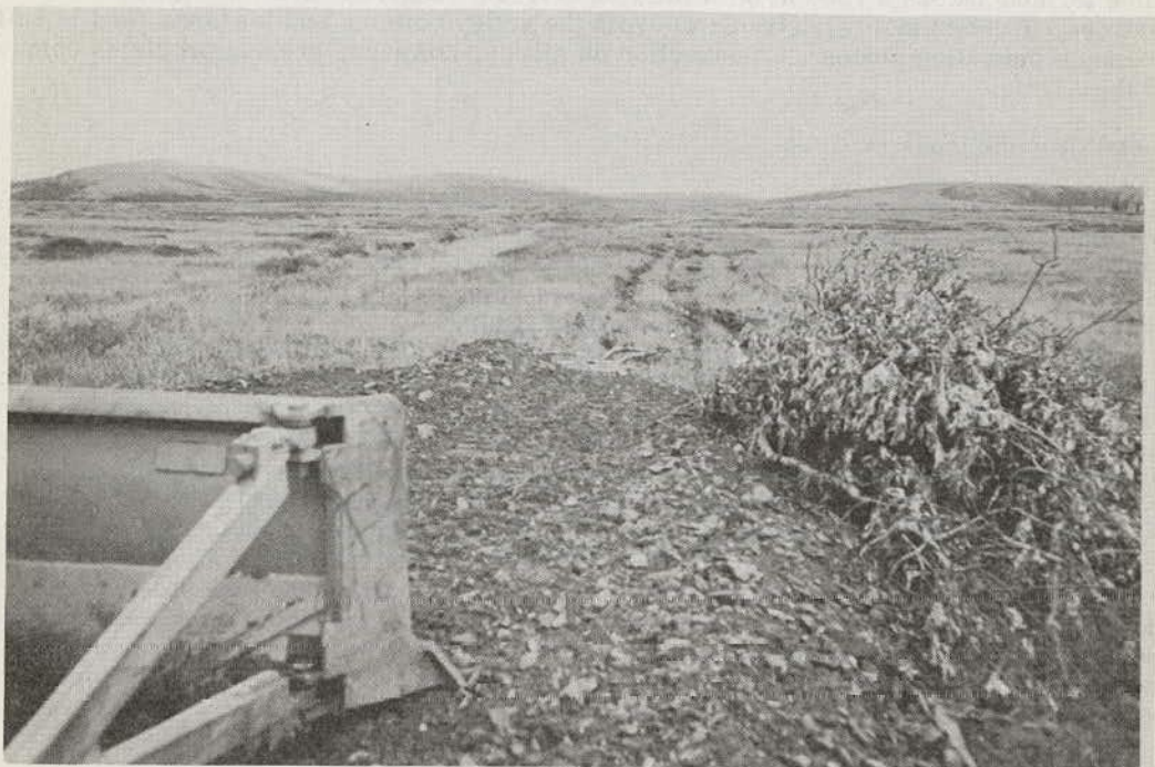
Figure 1. Road Construction in Area of Perennially Frozen Peat and Silt Near Council, Alaska. Gravel is Laid on Tundra without Disturbing Surface Vegetation.
