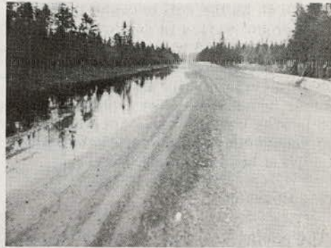
Figure 5. Granular Lift Necessary Before a Bituminous Surface Can Survive a Spring Breakup.
