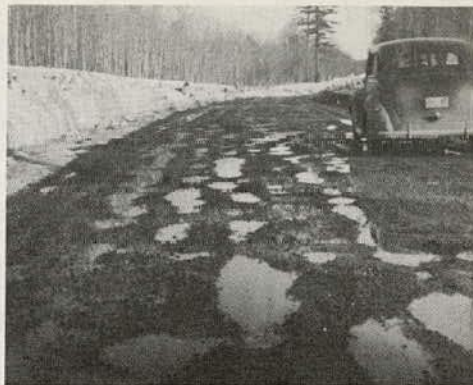
Figure 2. Snow Banks Preventing Proper Surface Drainage of Cross Section.
