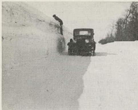
Figure 1. Snow Banks on the Highway Shoulder Indicating Drainage Problems to Come.
