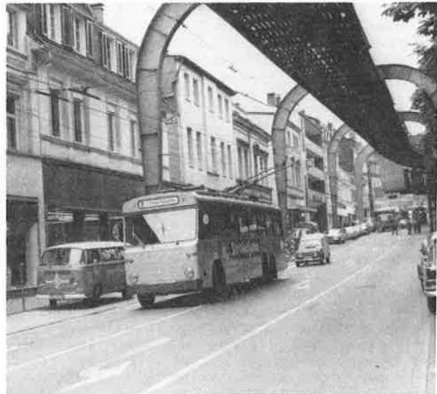
Three-axle trolley bus of Solingen, West Germany, under the Wuppertal Monorail, was built in 1972 and has auxiliary propulsion via a VW engine (photograph by J.P. Aurelius)
