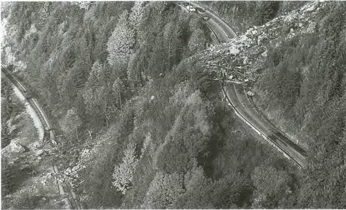
FIGURE 18-1 Railway and highway at Howe Sound, British Columbia, blocked by October 1990 rock fall that originated approximately 300 m above highway. DENISE HOWARD, VANCOUVER SUN
