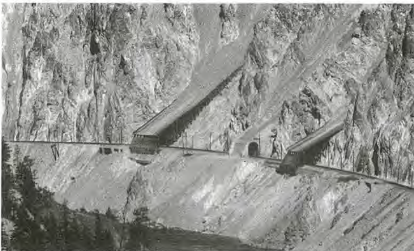
FIGURE 18-23 Rock sheds constructed with steeply sloping roofs that deflect rock falls over railway tracks. CANADIAN NATIONAL RAILWAY
