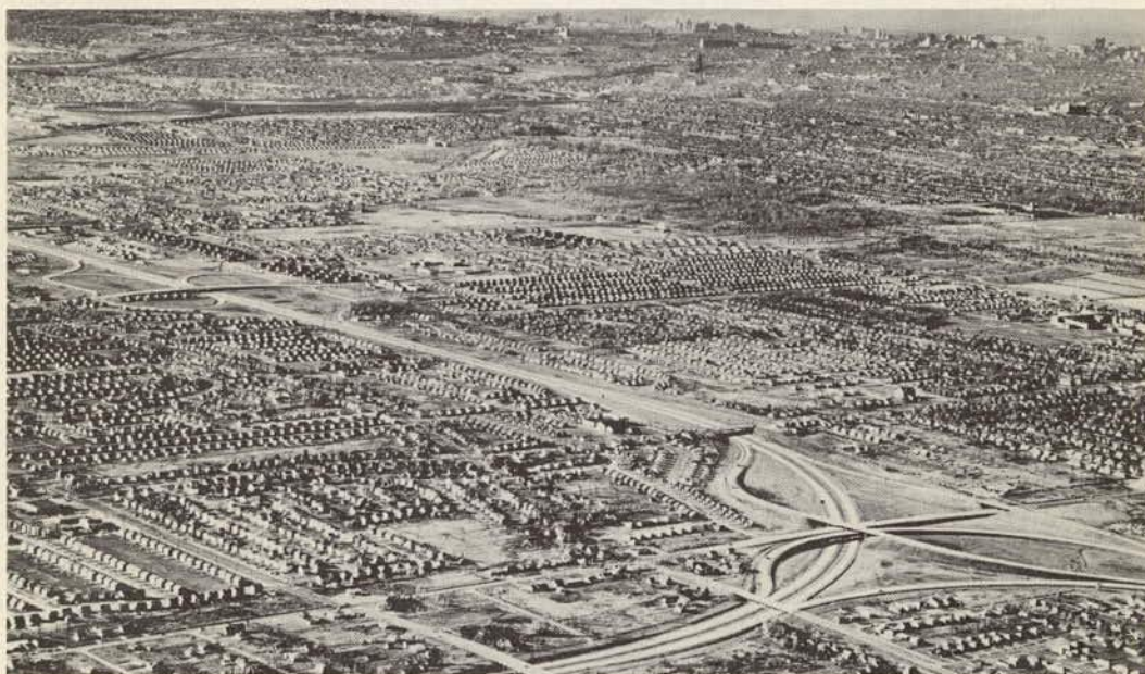
Before the New York State Thruway was built, this area east of Buffalo had developed only scattered residential tracts. The opening of the Expressway has opened up the entire area. It is reported that $50,000,000 in new building has been inspired by the thruway and that another $50,000,000 will be spent on capital outlay in this area when the the Thruway's Erie and Niagara sections are completed.
