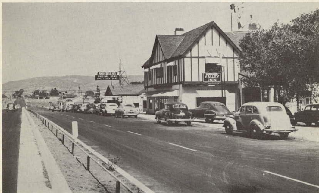
Property abutting the frontage road of this recently improved section of a California arterial constituted the subject of another land economics study.
