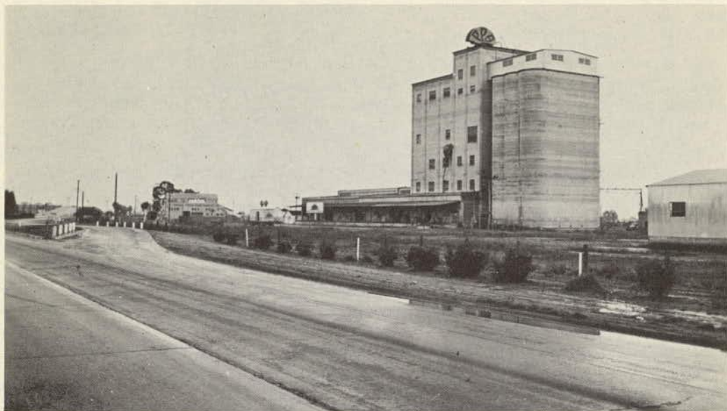
This grain elevator and warehouse, constructed adjacent to the Fresno Freeway in California, is typical of many similar uses along this highway of modern design. It has access to a county road to the rear. The economics of the Fresno Freeway have also been investigated.
