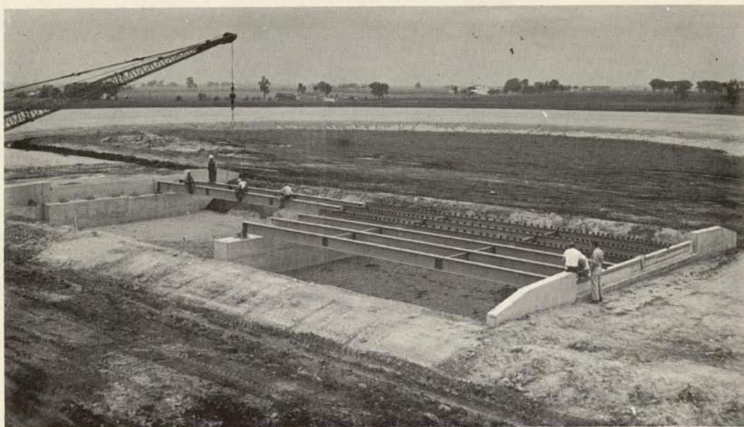
Figure 12. Erection of steel beams in Loop D.
