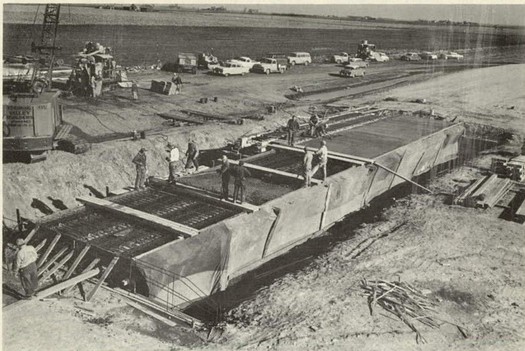
Figure 13. Casting of concrete slabs for prestressed concrete bridges.
