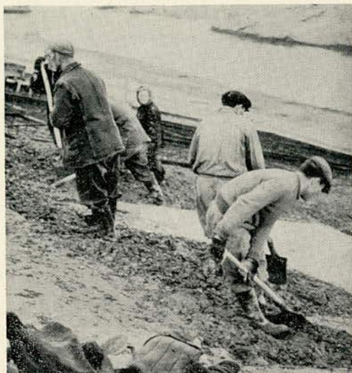
FIGURE 20 Hand placement of concrete in protective dike facings, Stalingrad Hydroelectric Station.
