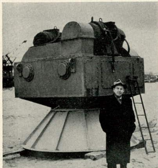
FIGURE 21 Unit with VP-160 vibrators for driving reinforced concrete cylindrical shell dolphins, Leningrad Harbor.
