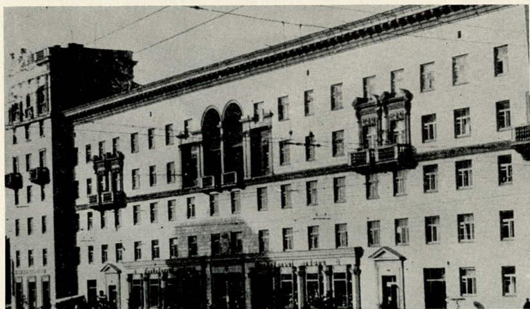
FIGURE 24 Foundations of this house in Zaporozhye were thermally underpinned (1955).
