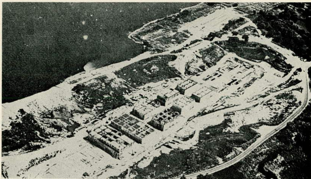
FIGURE 8 Foundation caissons under construction in the dry.
