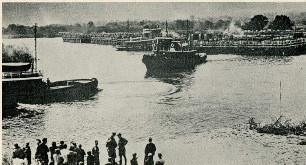
FIGURE 15 Towing first foundation caisson from construction basin.
