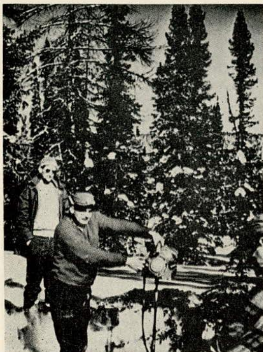
FIGURE 15 Acker Packsack portable diamond core drill.
