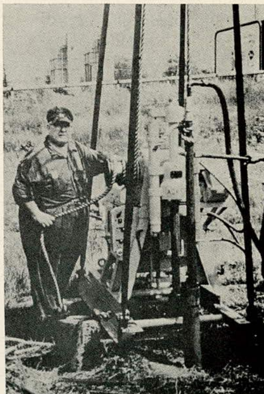
FIGURE 18 Skid-mounted Acker hydraulic feed Tereido.
