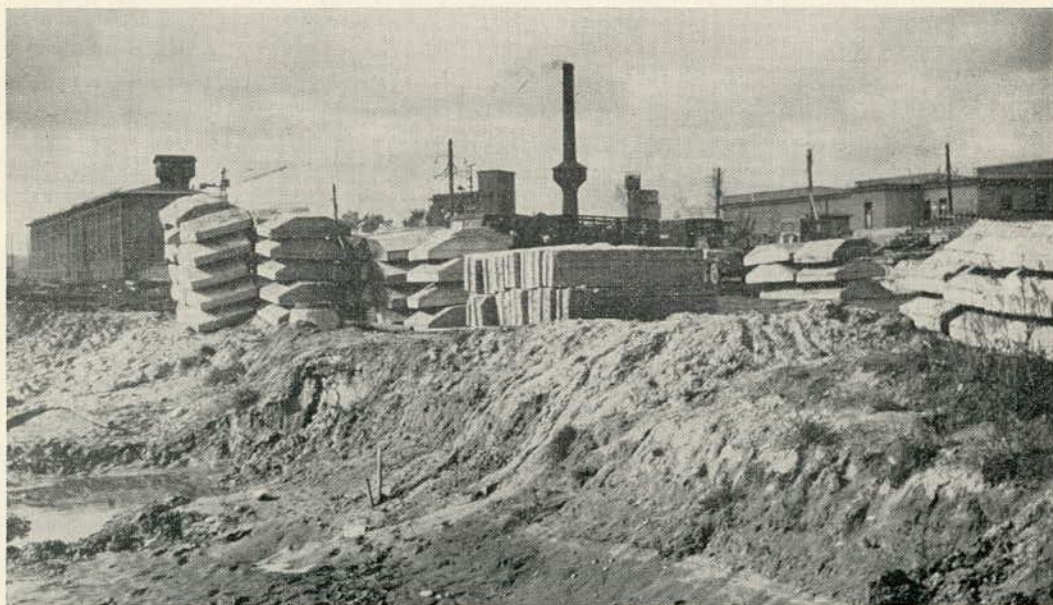
FIGURE 24 Precast footings for apartment buildings, Leningrad.
