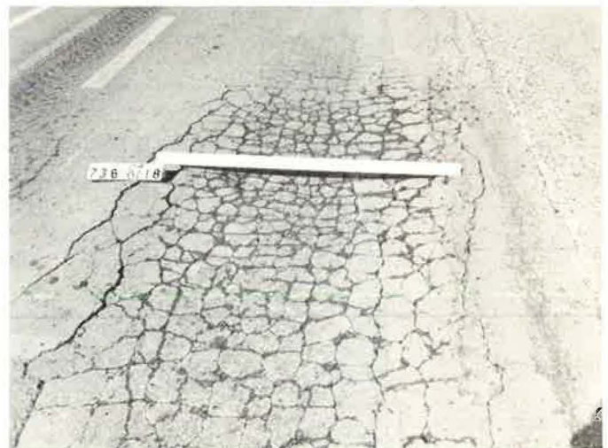
Class 3 cracking.
