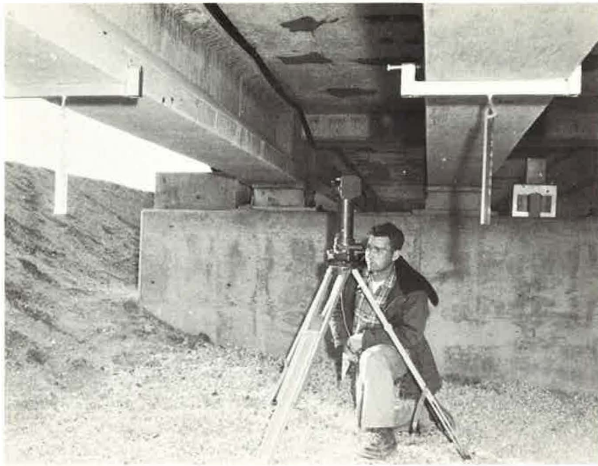
Figure 43. Brackets and scales for measurement of beam elevations.
