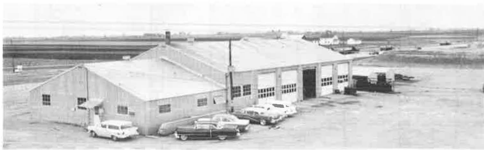
Figure 11. Vehicle maintenance garage.
