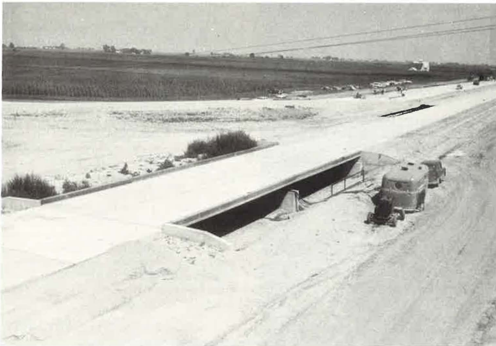
Figure 40. Set of four completed bridges.
