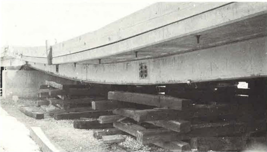
Figure 49. Bridge 1A at end of test.
