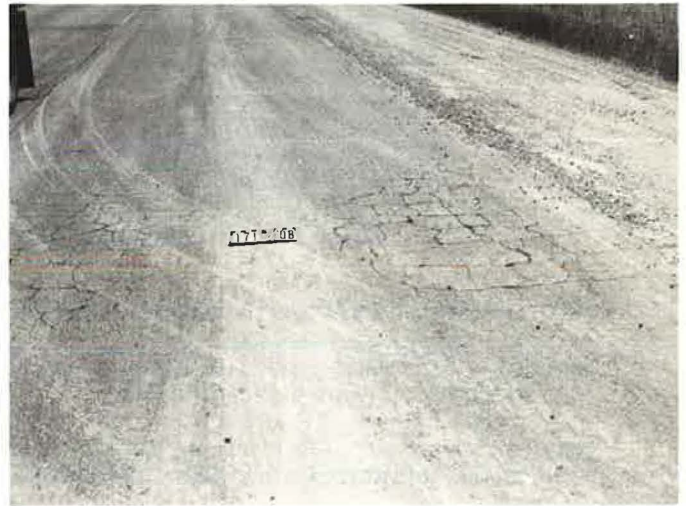
Class 2 cracking.
