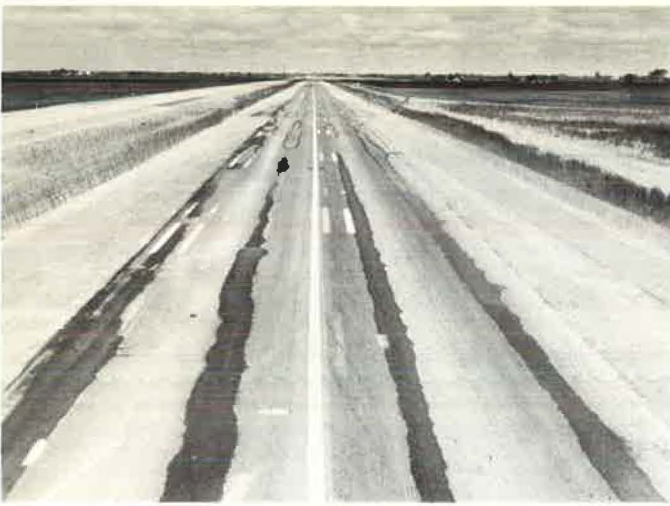
Evidence of longitudinal rutting, water in wheelpaths after a rain in a no-traffic period.
