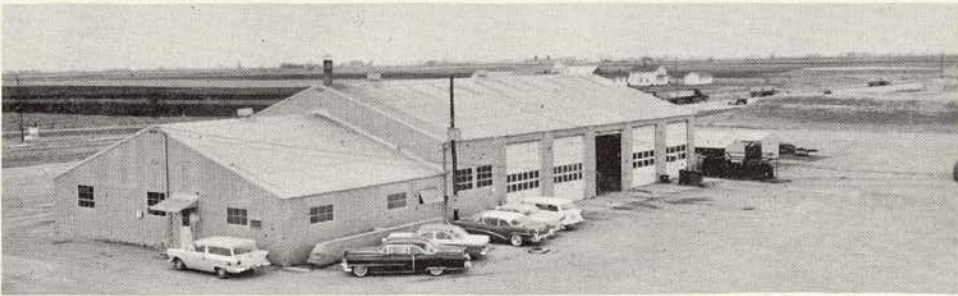
Figure 5. Vehicle maintenance garage.
