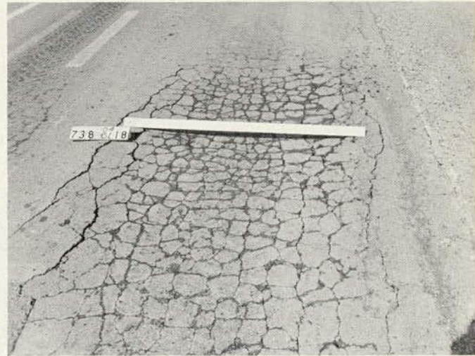
Class 3 cracking.
