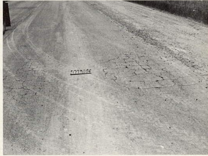
Class 2 cracking.
