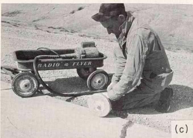
Figure 139. Successive stages in installation of strain gages on edge of pavement in traffic loops (see text for explanation).
