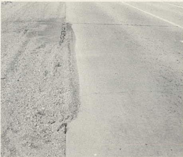
Typical pile of subbase material pumped from beneath pavement, showing change in gradation of material from fine to coarse in direction of traffic, toward reader.
