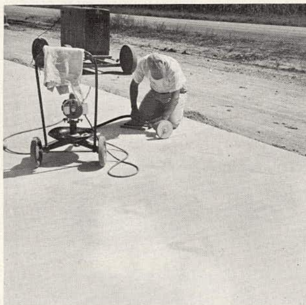
Figure 183. Two of the several steps in installation of strain gages in Loop 1.
